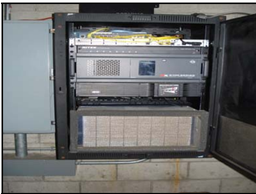
Photo 3 - Security Equipment Rack
