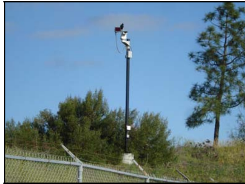
Photo 2 - Single pole with PTZ/IR
