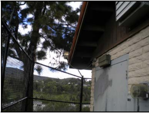
Photo 2 - Problem area on SW corner
