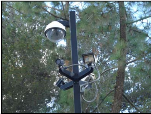
Photo 2 - Typical Pole Installation with CCTV/IR/MD
