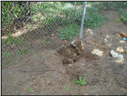
Photo 3 - Sample Breach Point
