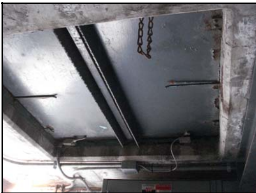
Photo 1 - Vault Hatch with sensors.
