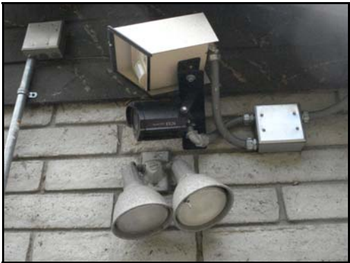
Photo 3 - Typical security equipment cluster
