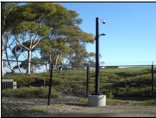
Photo 1 - CCTV on Pole
