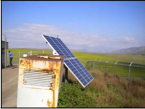
Photo 3 - View of Main Gate with PV and cabinet
