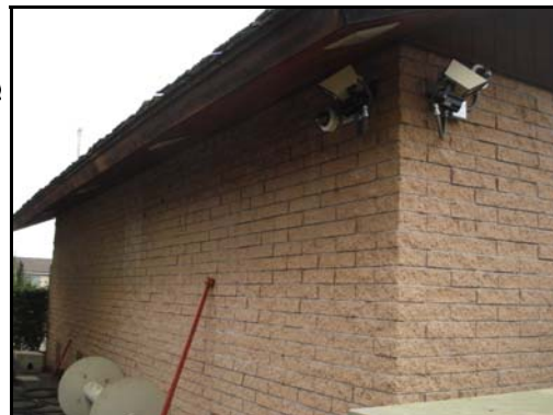
Photo 3 - Typical security cluster
