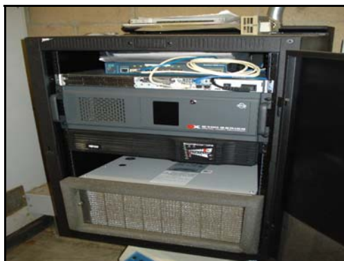
Photo 3 - Security Equipment rack
