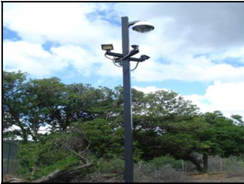
Photo 2 - Pole Installation with CCTV/IR/MD
