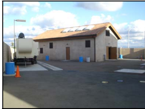
Photo 2 - Pump Station Building
