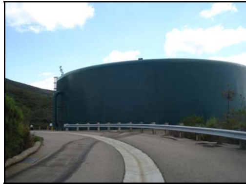
Photo 2 - View of Reservoir Tank with CCTV on top.
