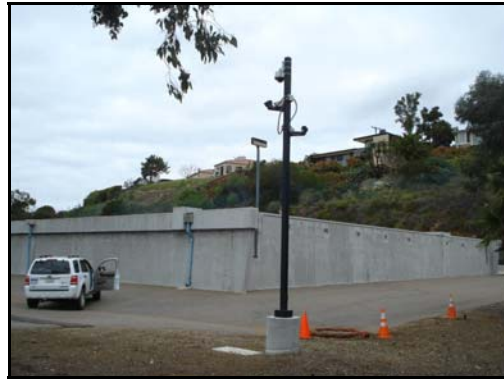
Photo 2 - View of security pole
