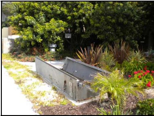
Photo 2 - General site view
