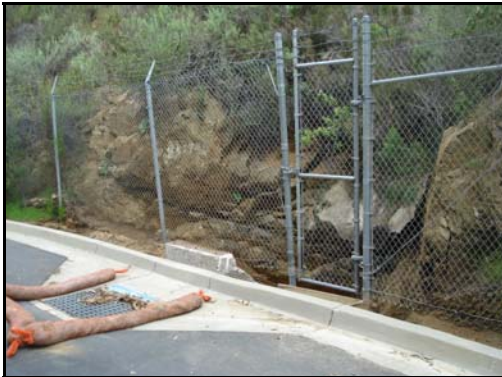
Photo 3 - Rear Ped Gate
