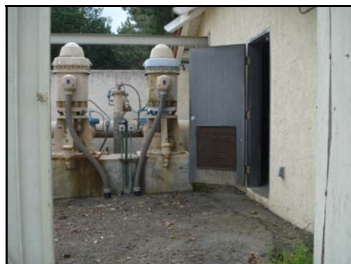
Photo 2 - Pumps and Building Entrance
