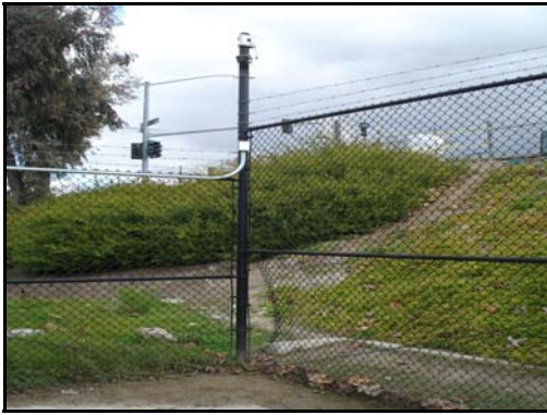
Photo 2 - NW Corner - Missing camera and breach location
