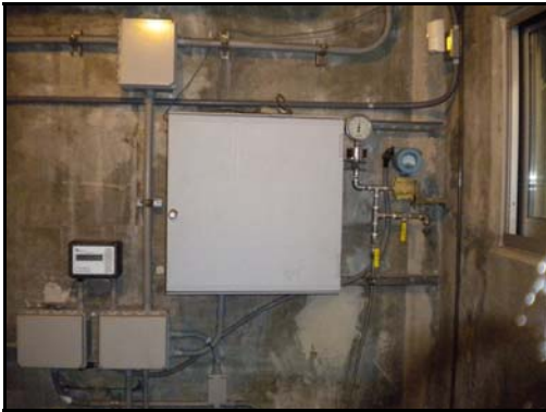
Photo 2 - View of vault Interior
