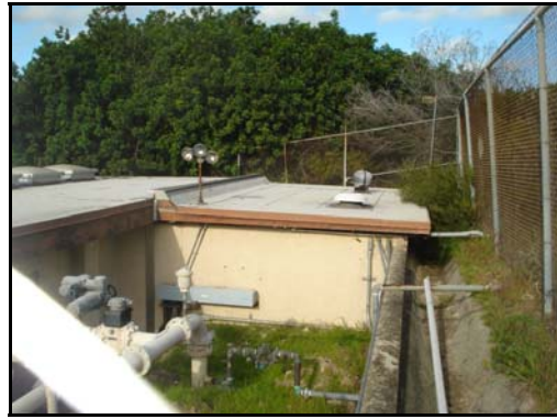
Photo 2 - Rear view of PS
