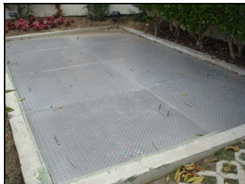
Photo 3 - Hatches in Public Area
