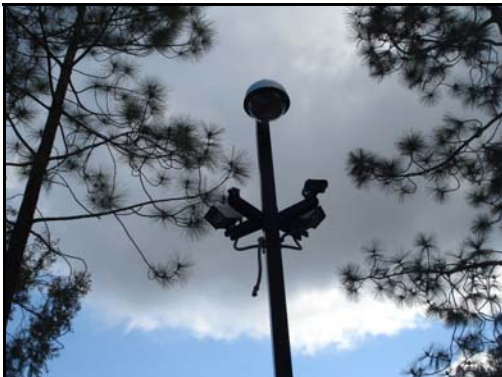
Photo 3 - Missing IR Unit
