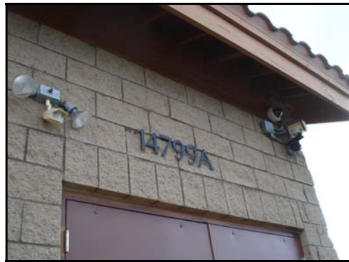
Photo 2 - Pump Station Building
