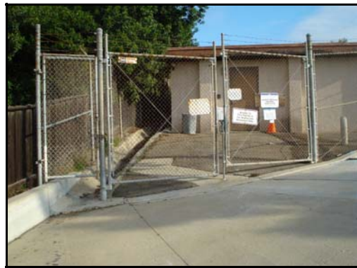
Photo 1 - Gate entrance to PS
