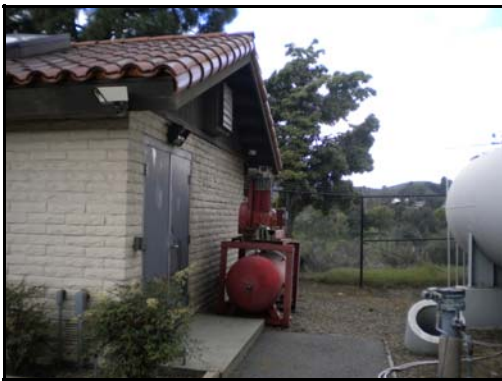
Photo 1 - North side of building
