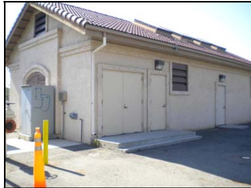
Photo 3 - View of South side of building
