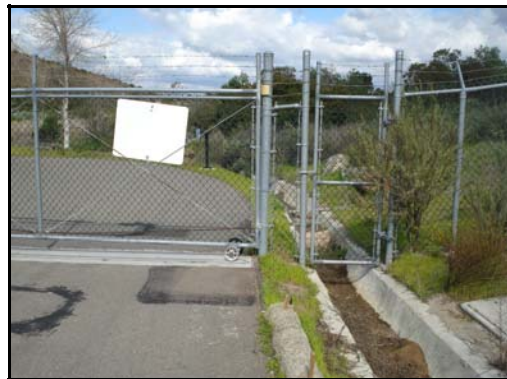
Photo 1 - Main Gate to Site
