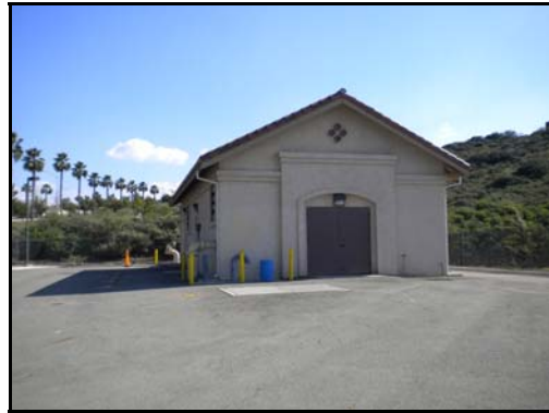
Photo 2 - View of North side of building
