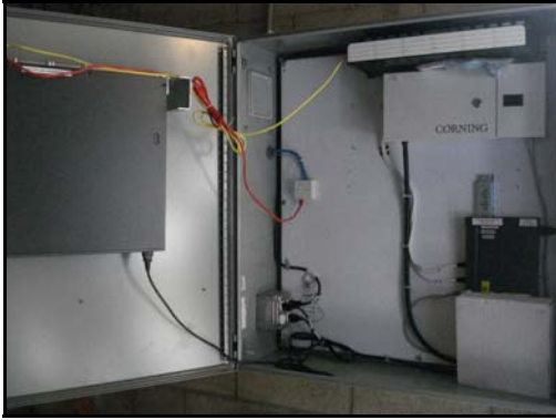
Photo 3 - Card Reader with access indicator
