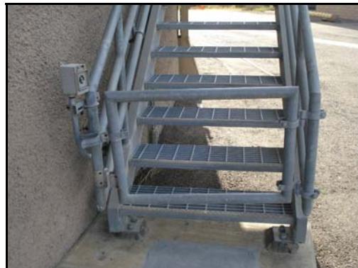
Photo 2 - Stair to Reservoir Roof
