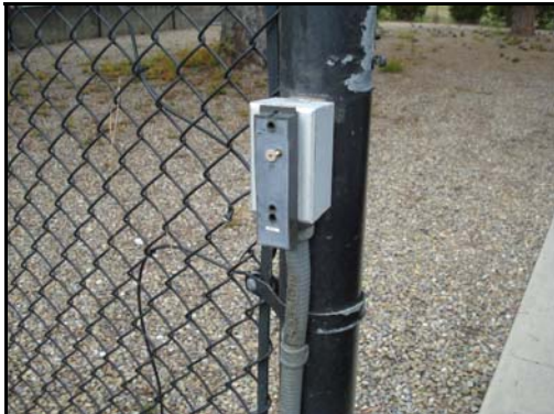
Photo 2 - Broken card reader at ped gate
