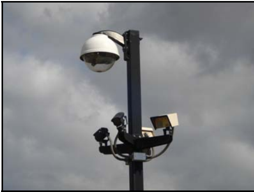
Photo 2 - Typical Security Pole Installation
