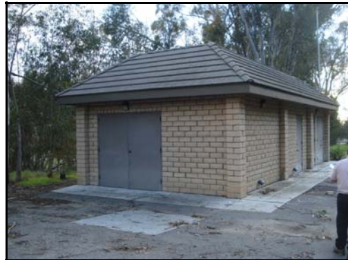
Photo 1 - Pump Station Building
