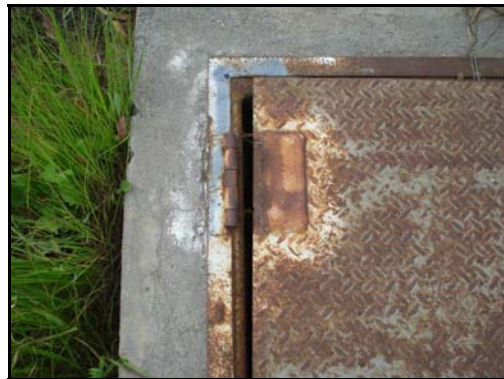
Photo 3 - Rusted Hatch Lid
