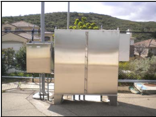
Photo 3 - Outdoor Security Cabinet
