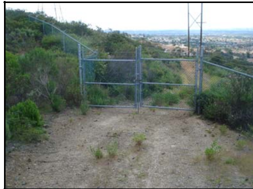
Photo 1 - Sample Perimeter Gate
