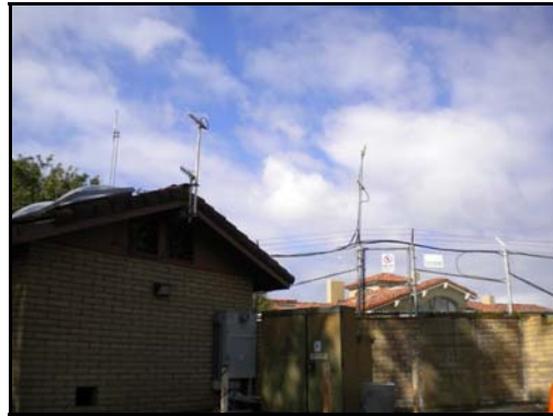
Photo 2 - Existing Antennas at Site
