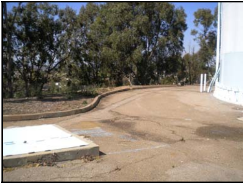
Photo 3 - Interior of Site
