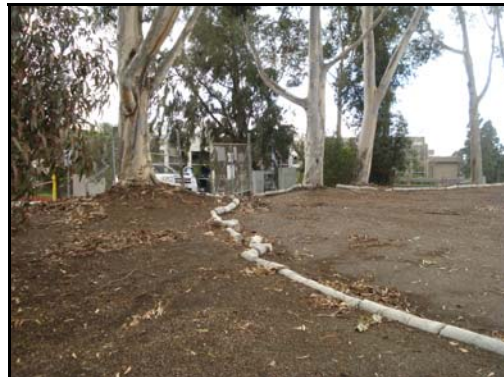
Photo 3 - General Site Conditions
