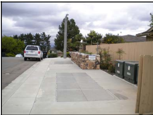
Photo 1 - View of vault site
