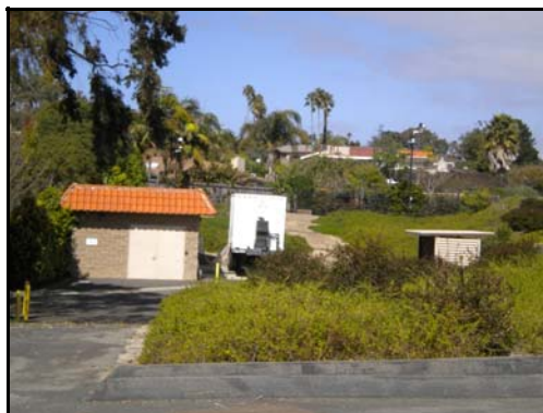
Photo 1 - Pump Station Building
