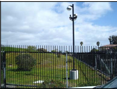
Photo 1 - Main Entrance CCTV/Motion Detector
