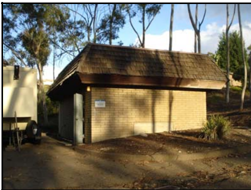
Photo 1 - Pump Station Building
