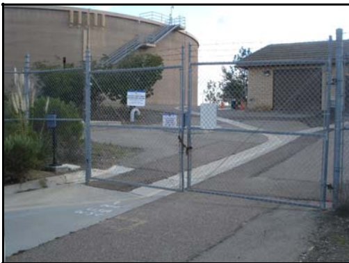
Photo 1 - Entrance to Pump Station Building
