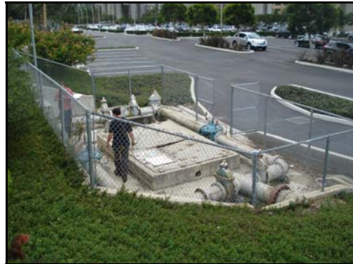
Photo 3 - Opposing view of site
