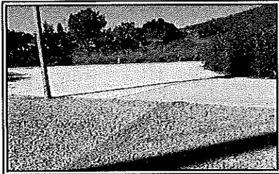
*An accessible path of travel to and from the skate park to the accessible parking spaces and loading zone is required by the 2010 ADA Standards. Portions of the walkways' and sidewalks' current cross slopes exceed 2%.*
