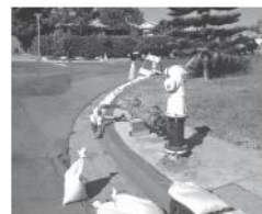
Temporary water pipeline connections ensured water reliability during construction along La Paz Drive.
