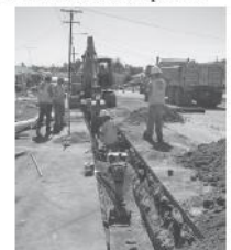
Crews work to replace old cast iron pipes with new pipes.
