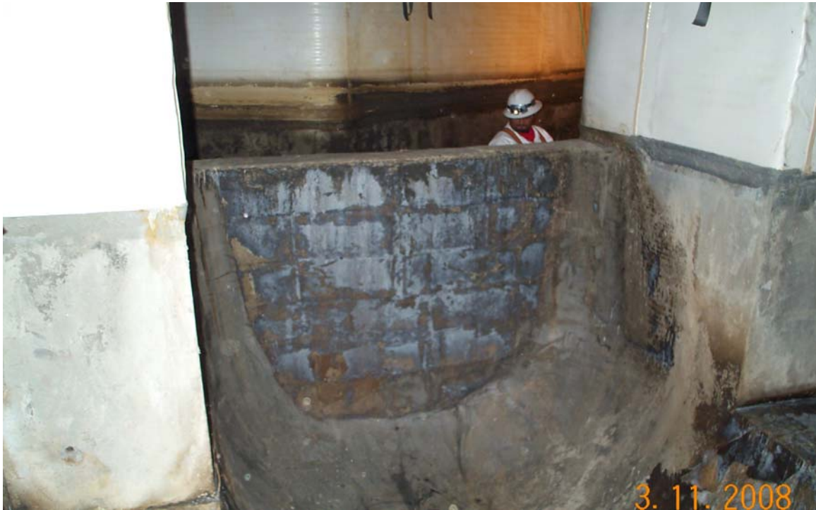
Install Arrow-Lock at newly constructed concrete wall
