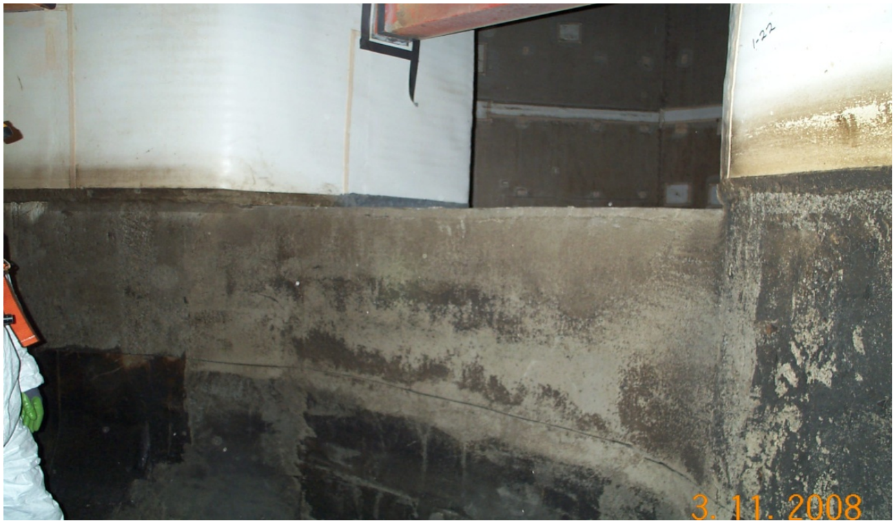
Install Arrow-Lock at channel wall
