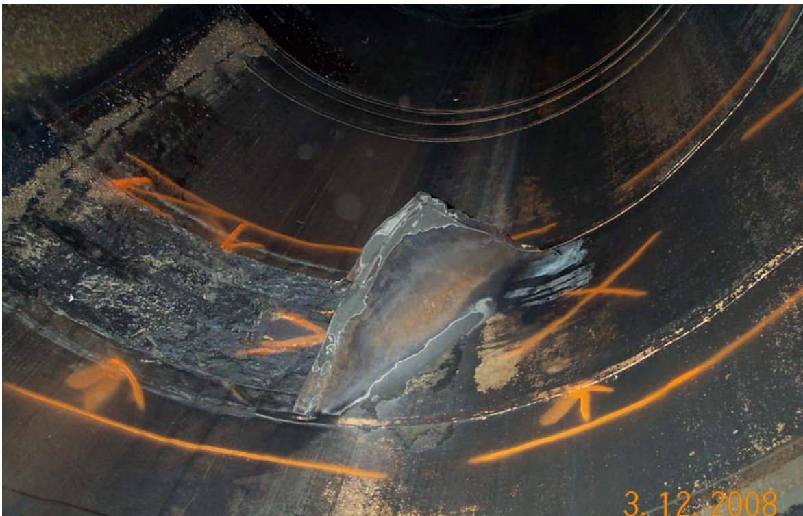
Remove and replace damaged liner at 84-inch pipe
