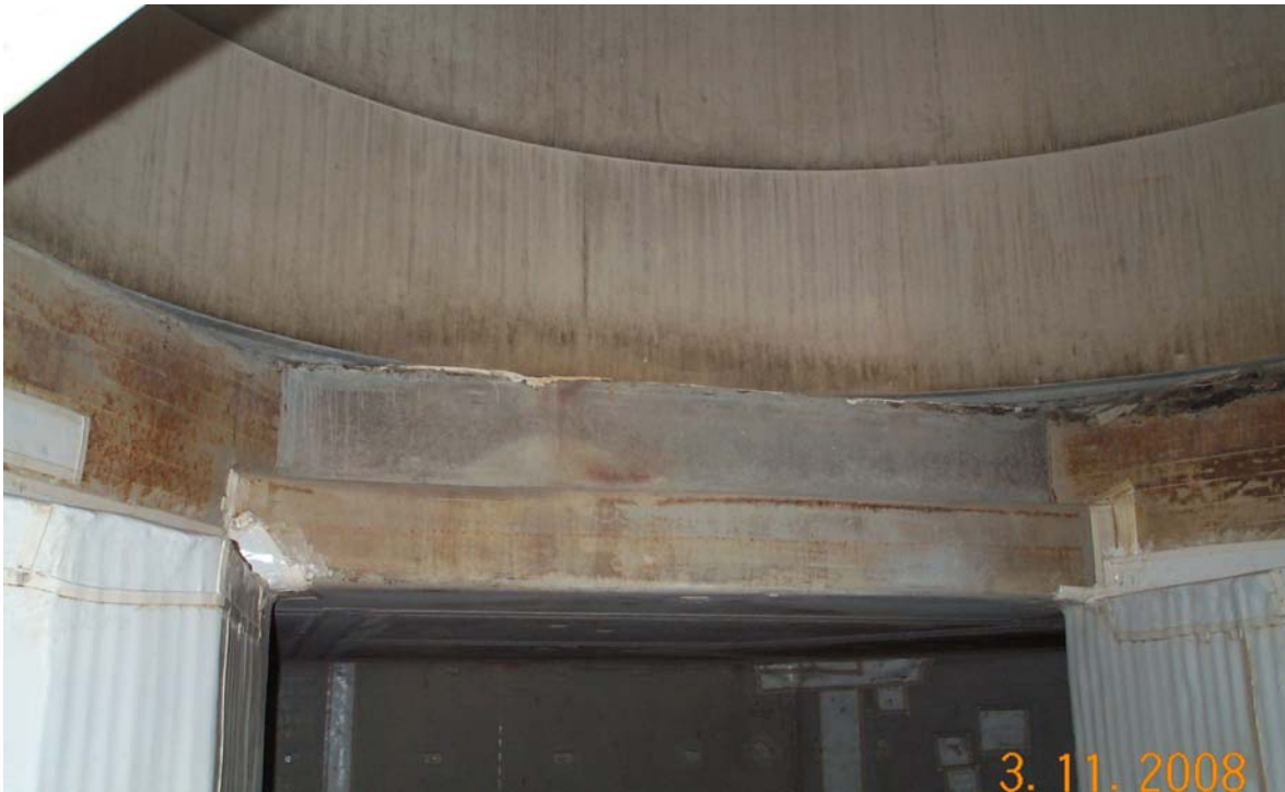
Install Arrow-Lock at concrete beam
