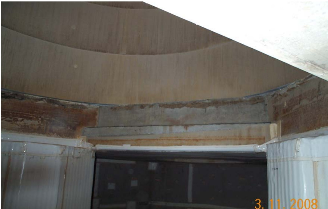
Install Arrow-Lock at concrete beam
