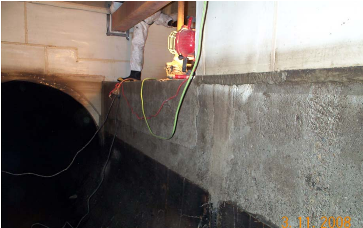
Install Arrow-Lock at channel wall
