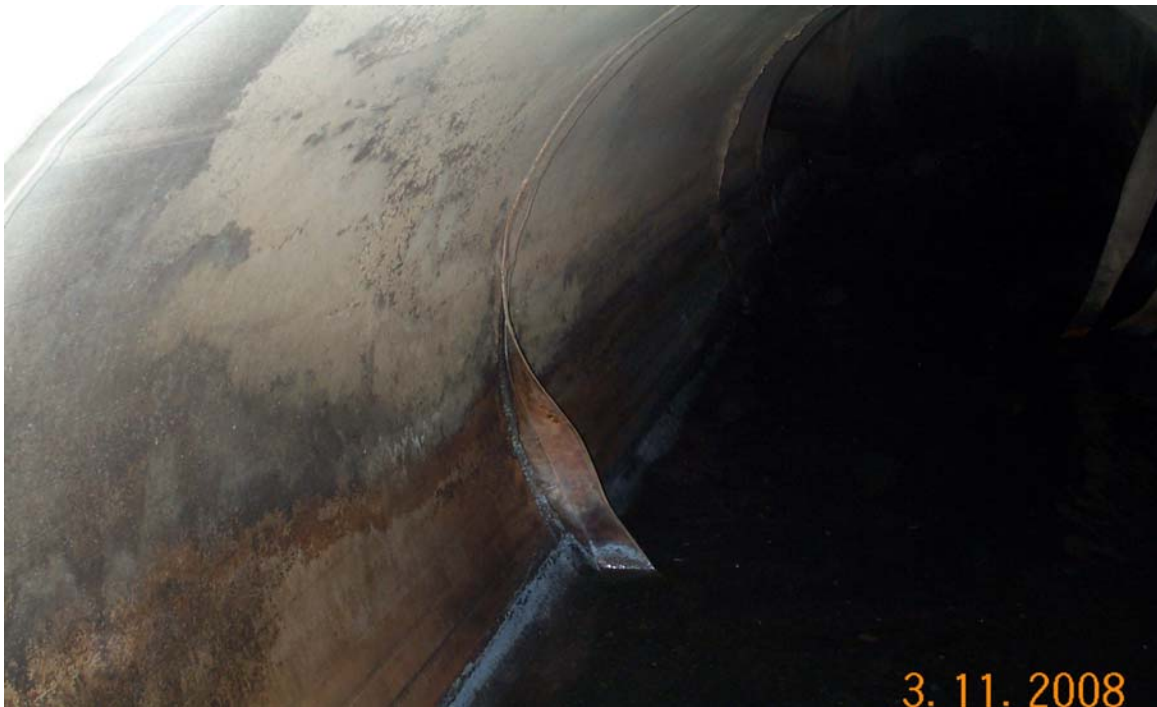
Remove and replace damaged liner at 84-inch pipe
