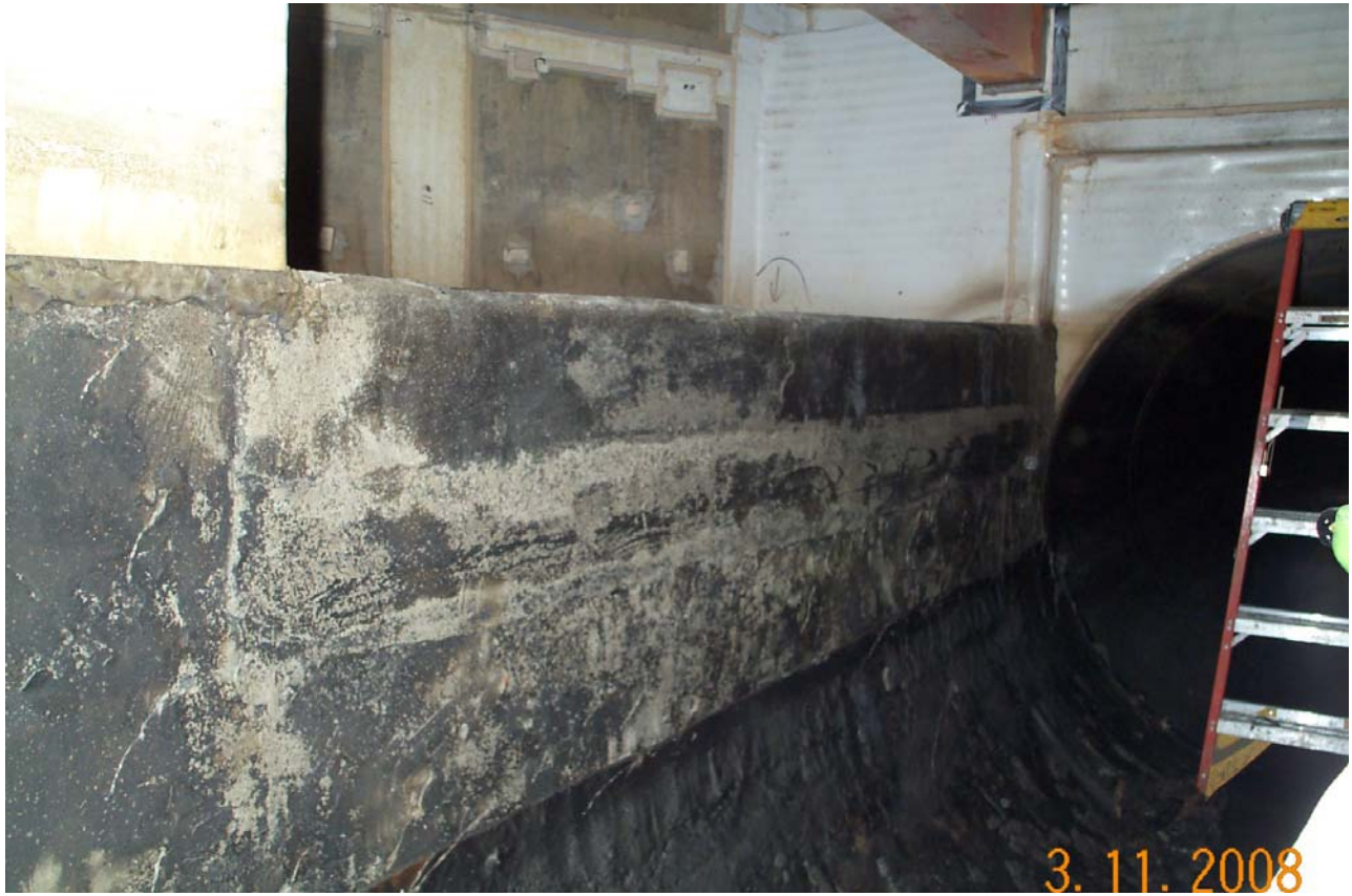
Install Arrow-Lock at channel wall
