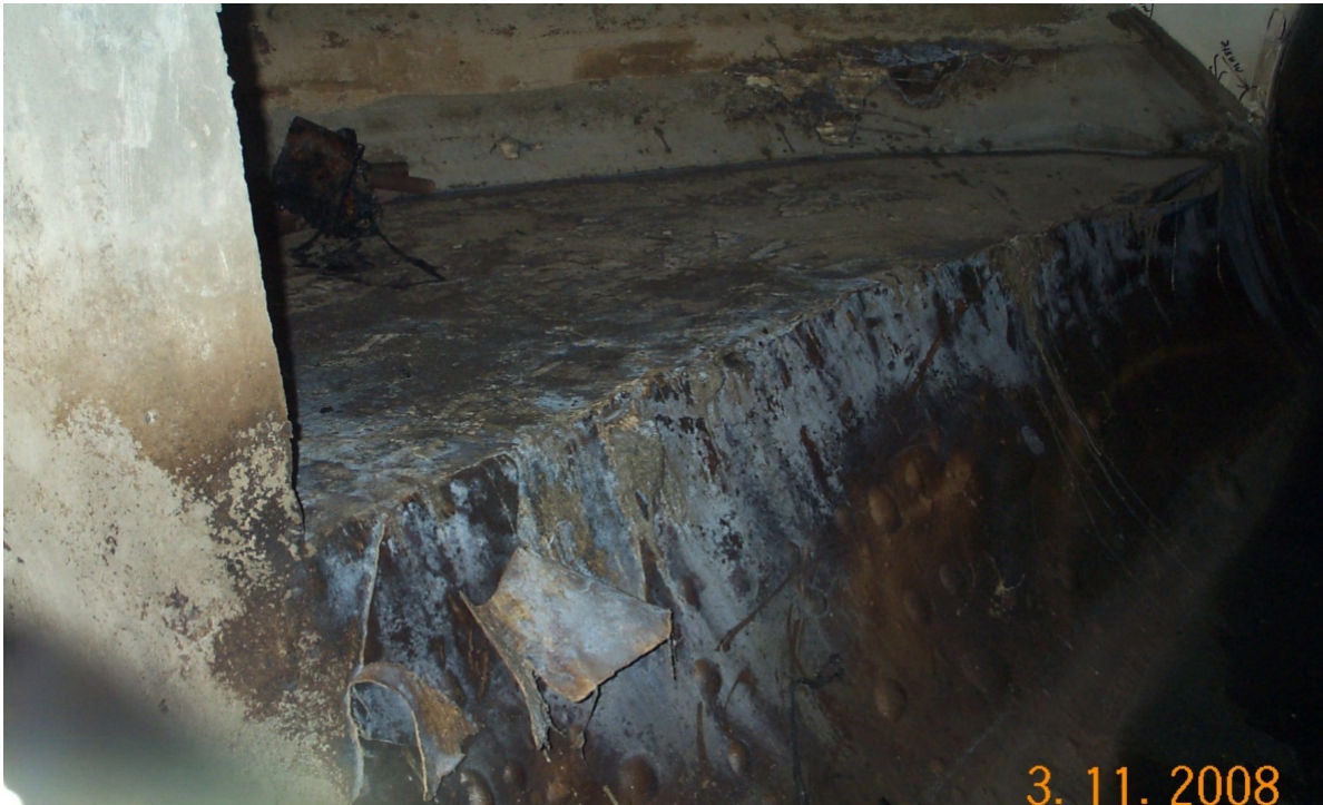
Remove existing spray liner and install new Arrow-Lock at side channel
