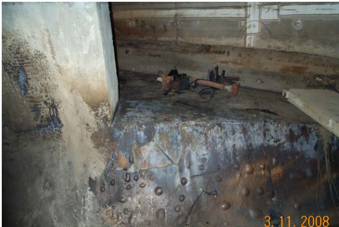
Remove old spray liner and install new Arrow-Lock
