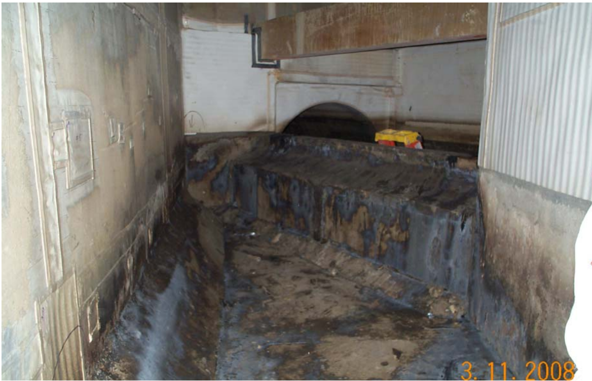
Install Arrow-Lock at concrete spillways
