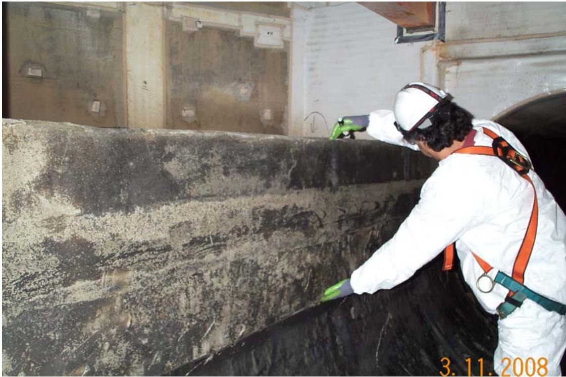
Install Arrow-Lock at concrete wall
