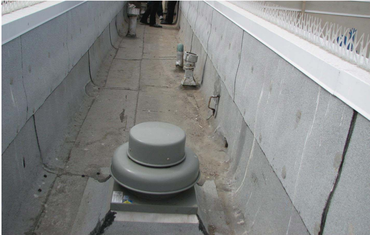
FIGURE 5: VENTILATION FANS ON FLAT ROOF SECTIONS
