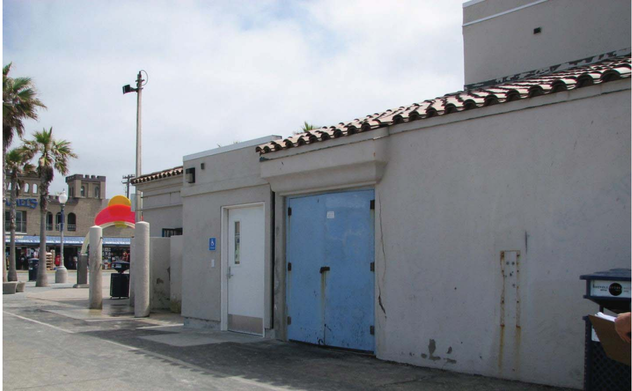
FIGURE 21: ELECTRICAL ROOM DOORS, PARK & REC RESTROOMS & SHOWERS
