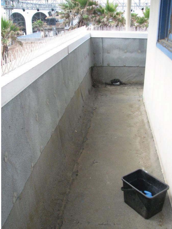
FIGURE 7: EAST SIDE OF TOWER
