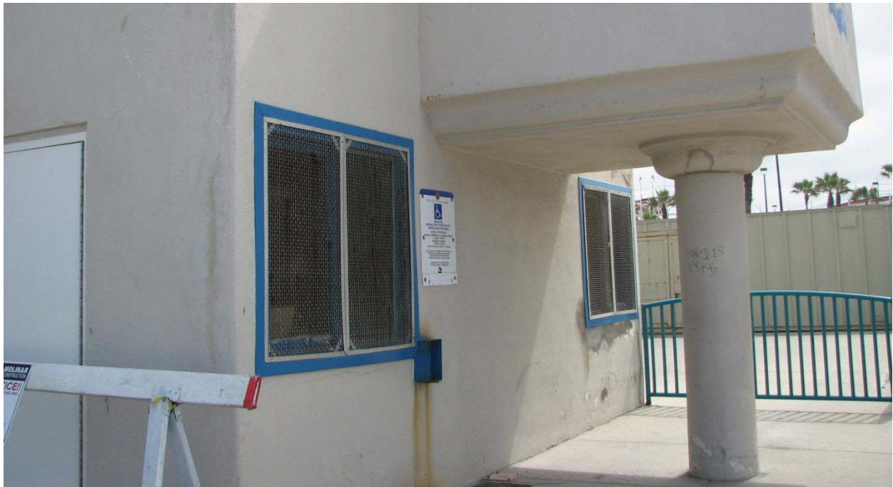
FIGURE 18: METAL WINDOW CAGES ON 1 ST FLOOR WINDOWS
