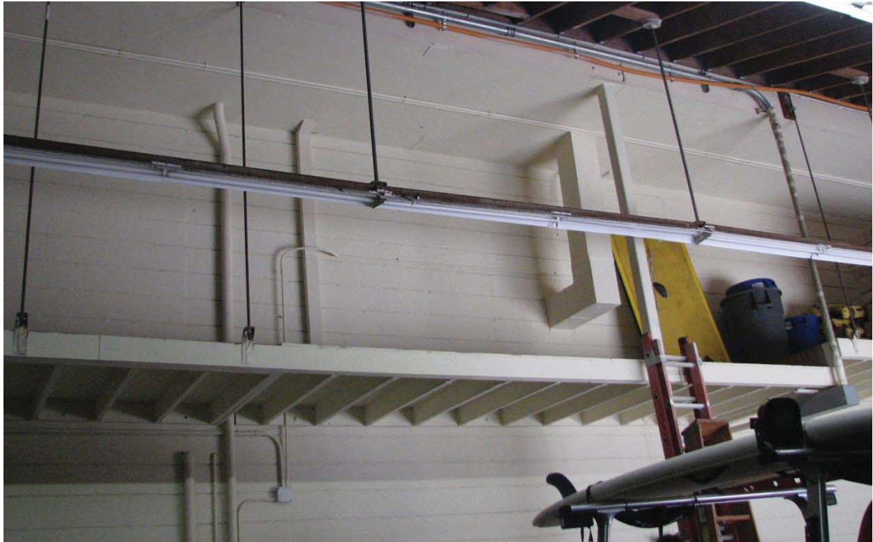
FIGURE 19: VENTILATION DUCTS LEADING TO ROOF
