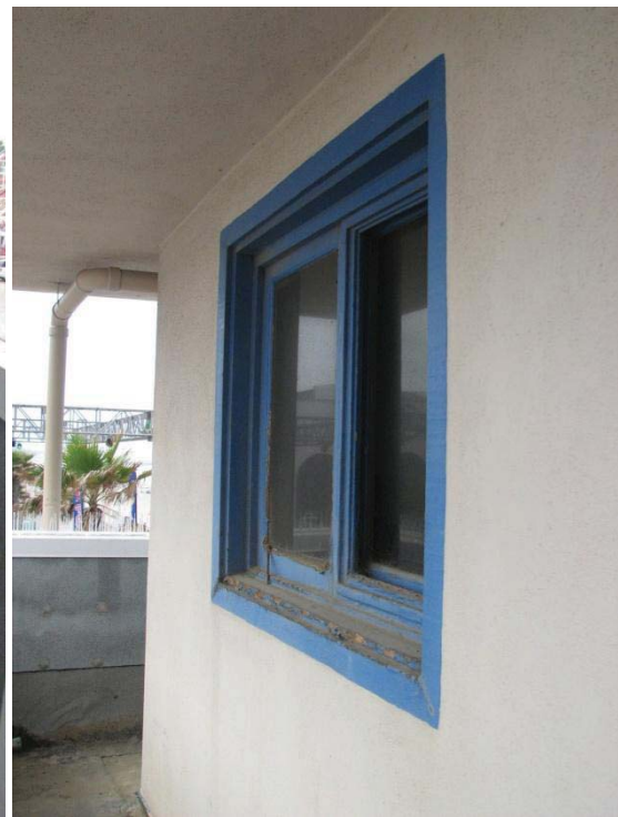
FIGURE 10: EAST SIDE WINDOW ON TOWER
