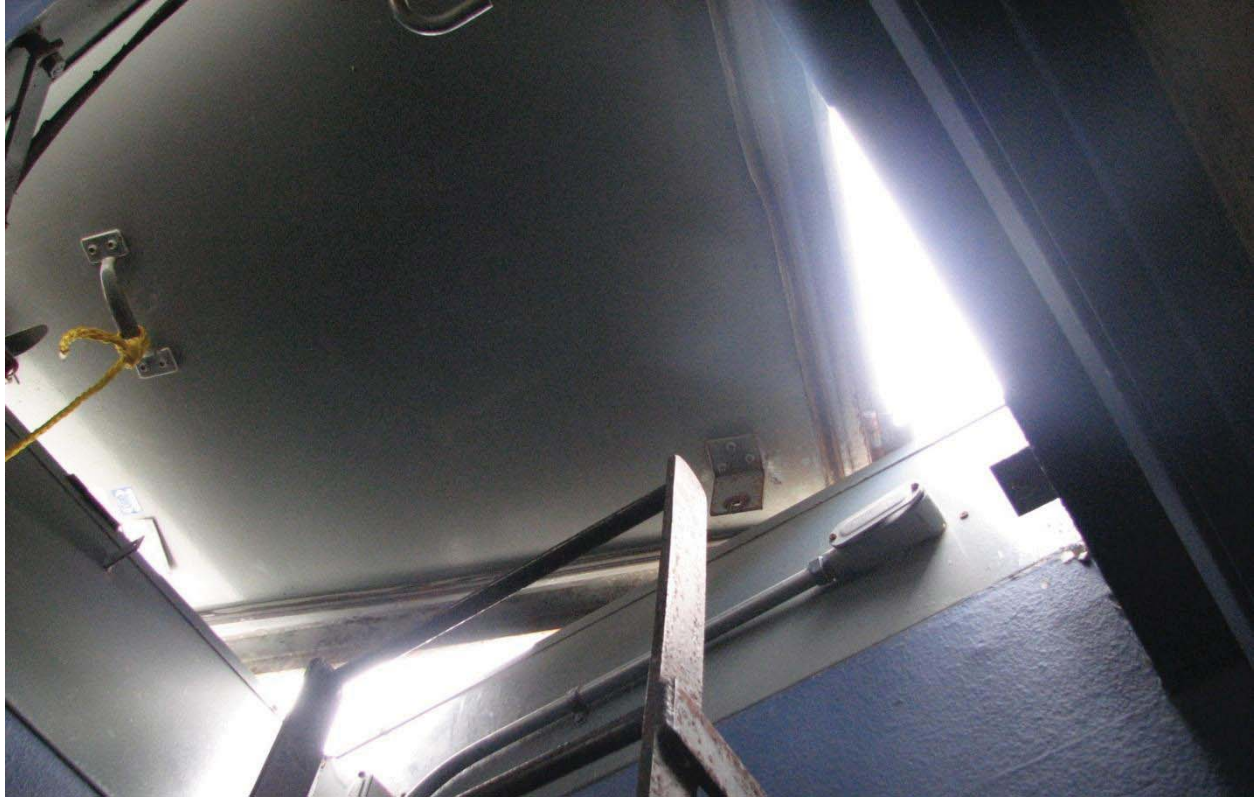
FIGURE 11: BROKEN ROOF ACCESS HATCH TO TOWER ROOF
