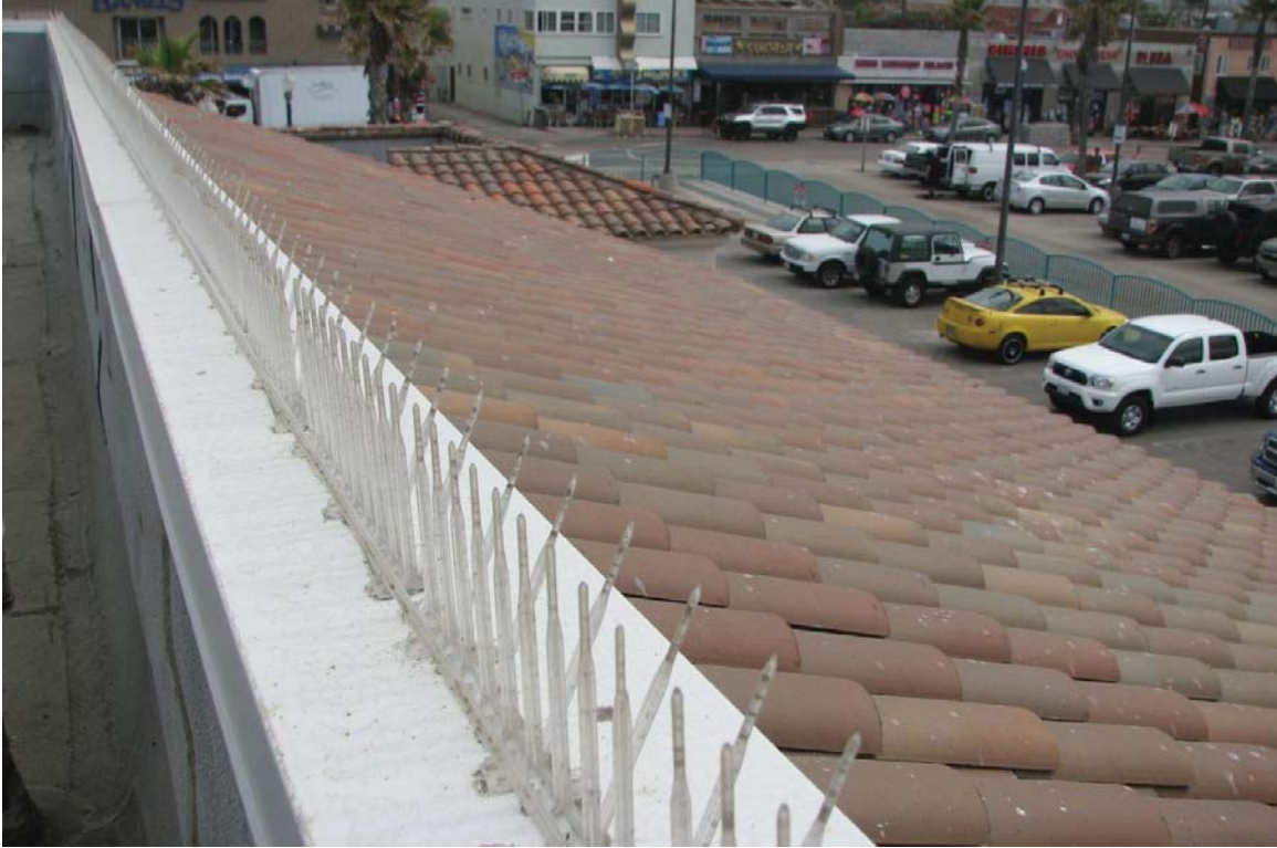
FIGURE 3: TILED ROOF ON THE EAST FACING ROOF
