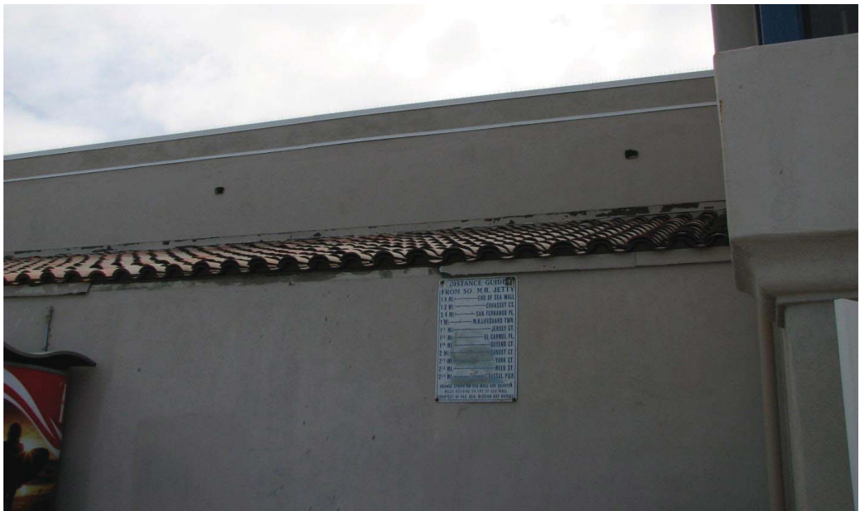
FIGURE 20: WEST SIDE OF LIFEGUARD STATION
