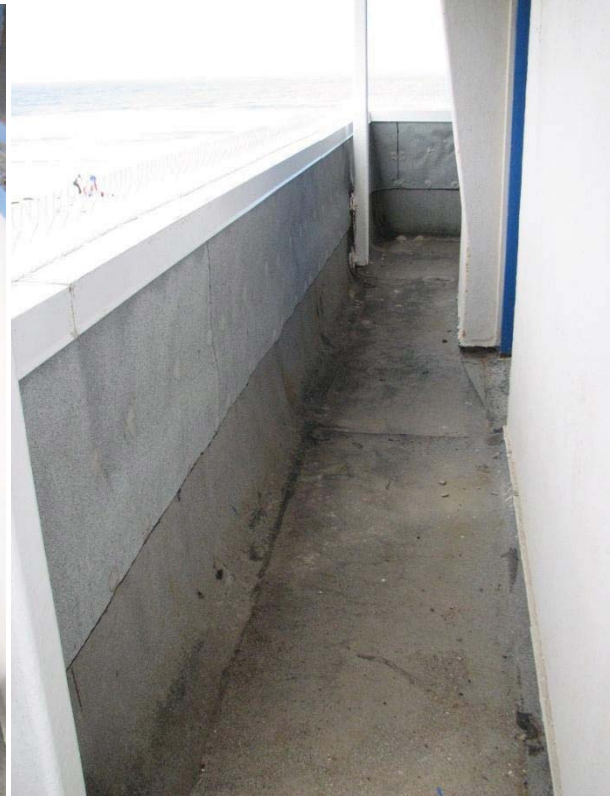
FIGURE 8: SOUTH SIDE OF TOWER
