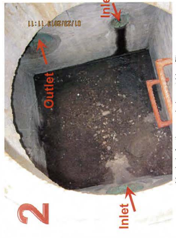
Manhole for the manhole cartridge filters
