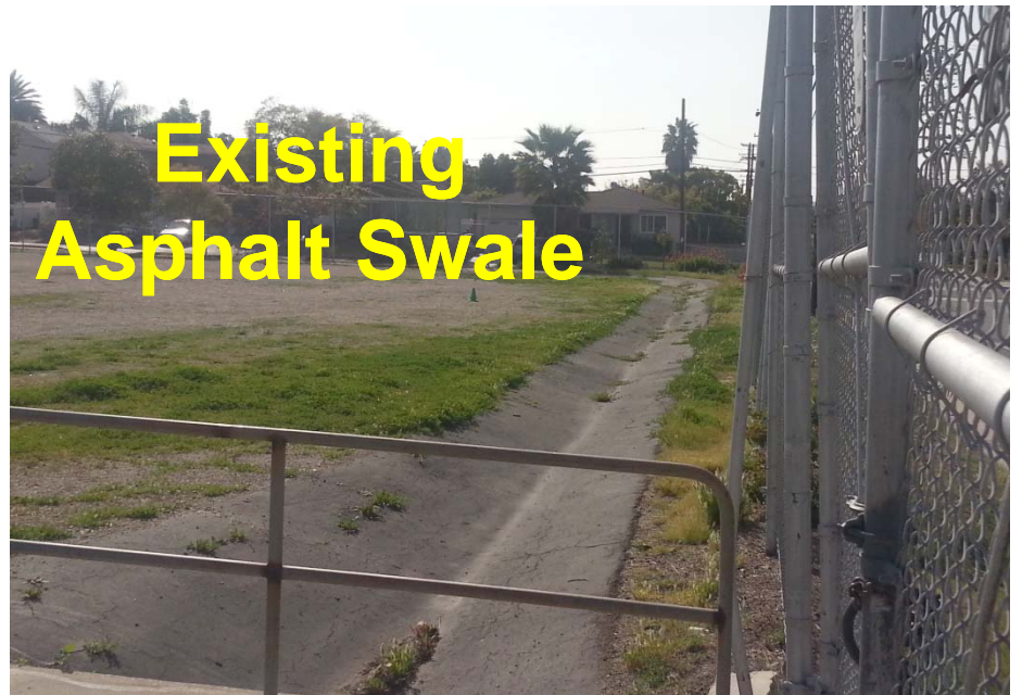
Existing Asphalt Swale
