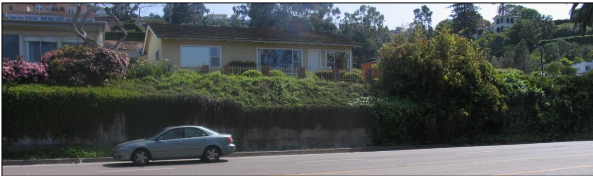
Picture 1345 - Concrete Block Retaining Wall near R.O.W.
