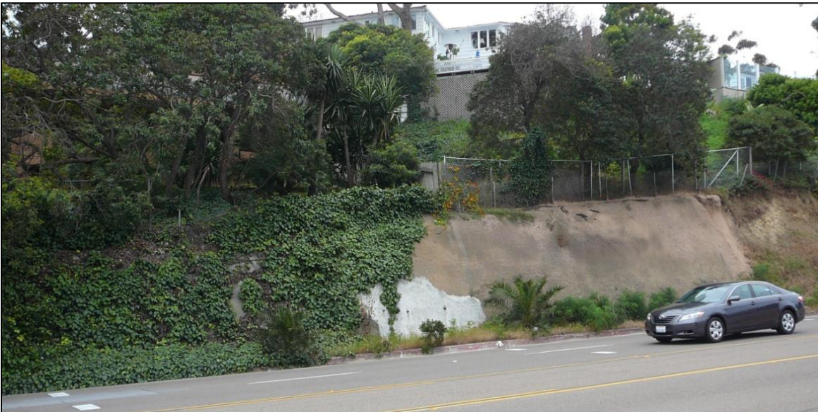
Picture 3943 - Station 19+00 South Slope with Existing Gunite Retaining Wall
