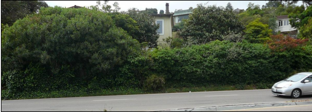
Picture 9 - Existing Wall at Approximate Station 45+50
