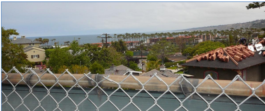
Picture 3916 - View over Fence at Station 42+00
