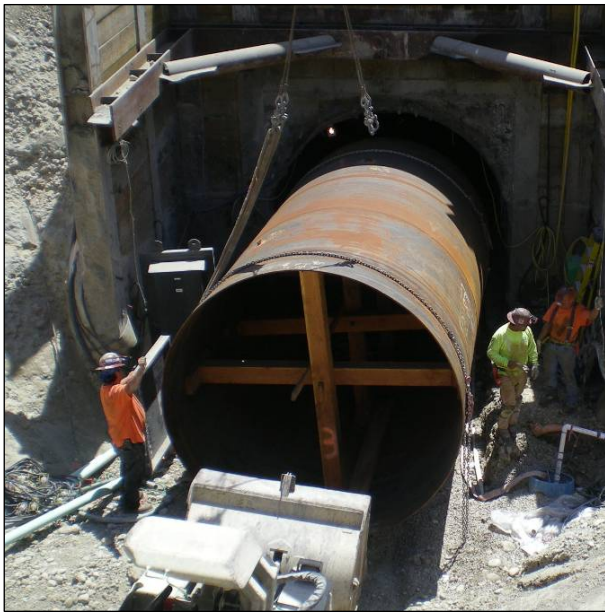
Pipeline carrying untreated water into the plant is in a tunnel under floc-sed basin 3.
