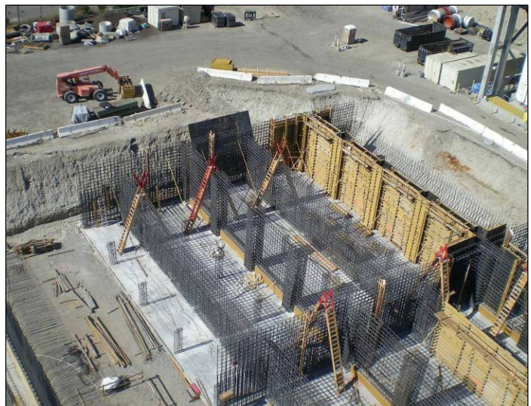
Flocculation-Sedimentation Basins 7 and 8.
