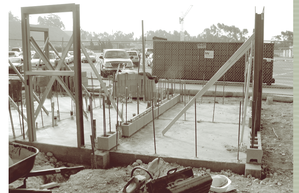
Contractors working to install new restroom facility at Lake Miramar.
