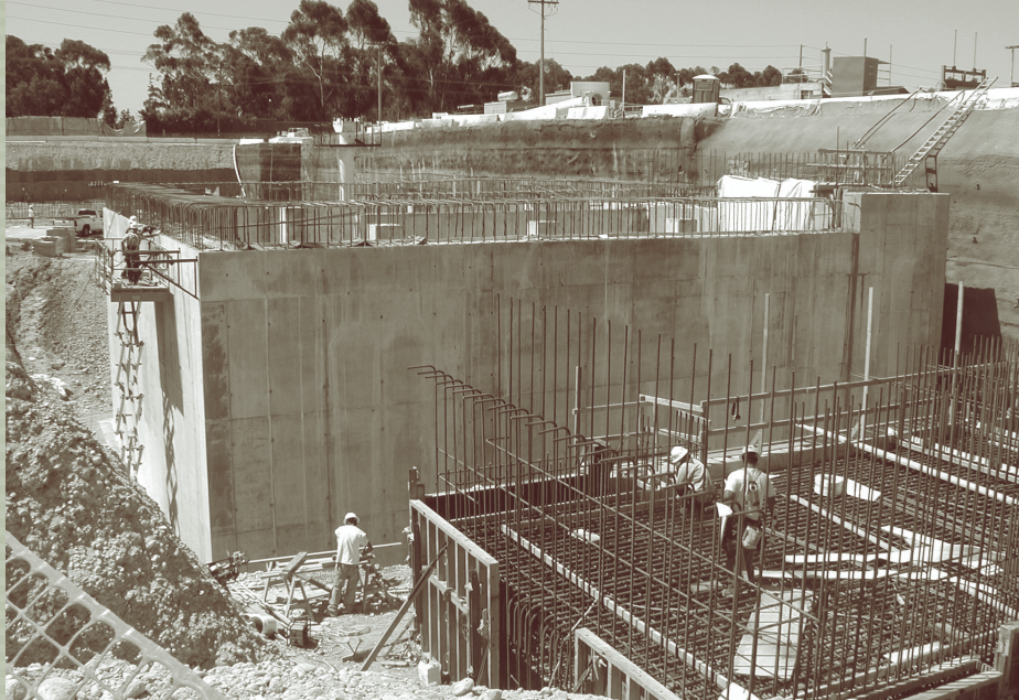
Concrete work at the new equalization basin.
