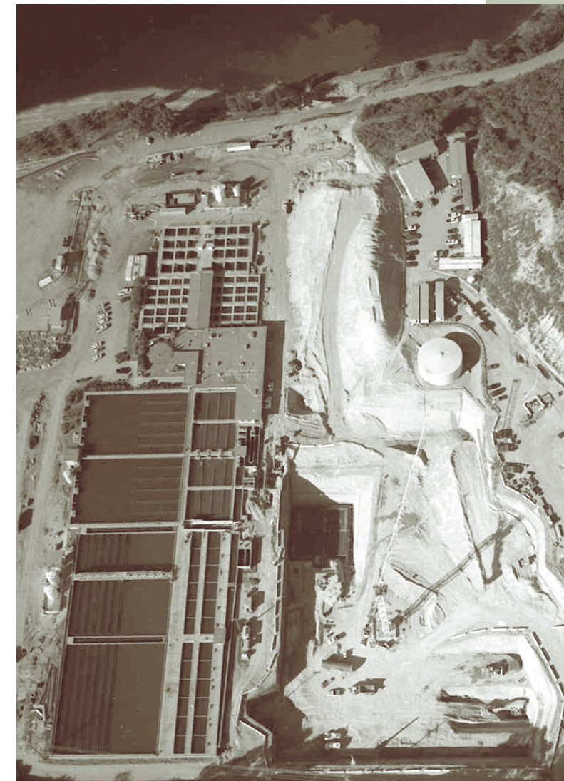
Aerial of Miramar Water Treatment Plant
