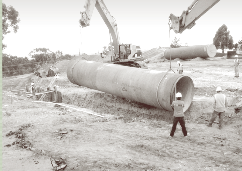
Contractors work side by side to install this 20' section of 90" pipe.
