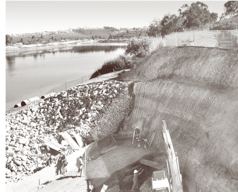
Contractors trench for the installation of a 108-inch pipe.
