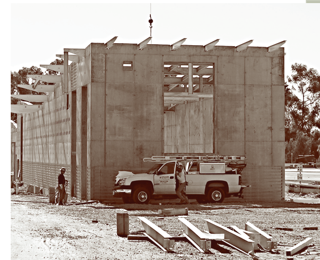
The first set of structural steel roof beams go up at the chlorine building.
