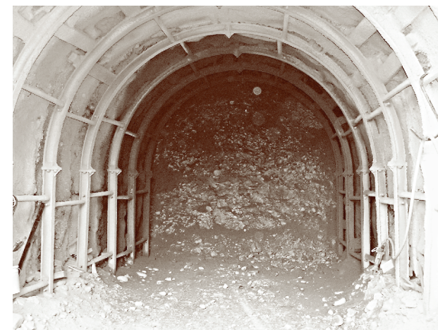
A 10-foot pipeline will be inserted into this 12-foot tunnel, to connect the effluent water with the new filters.
