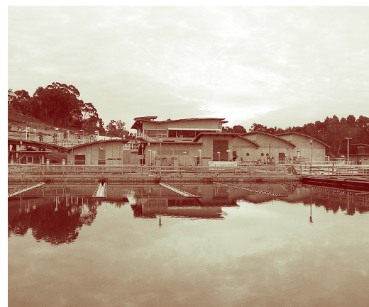
The new administration building and other structures, seen from the rear across the existing flocculation-sedimentation basins.
