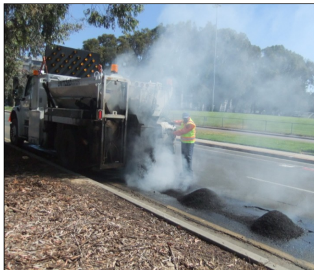
City crews recently spent a week repairing potholes throughout District 1.
