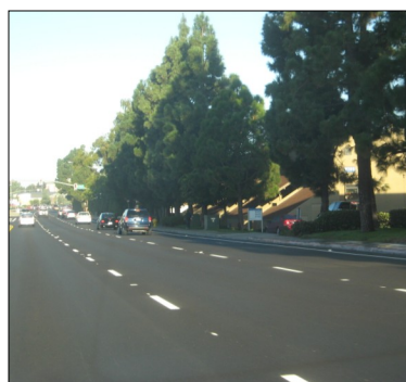
There is now smooth driving along Genesee Avenue between Fez Street and Campus Point Drive.
