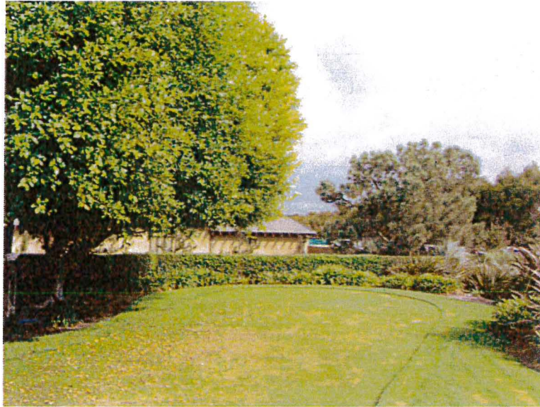
Looking at north elevation
