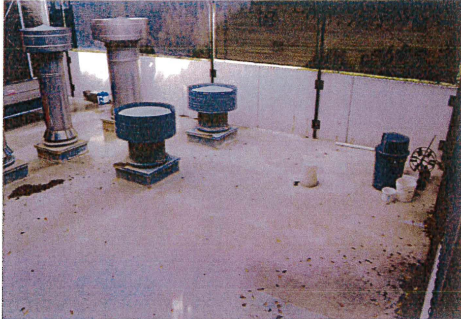
Looking at equipment location
