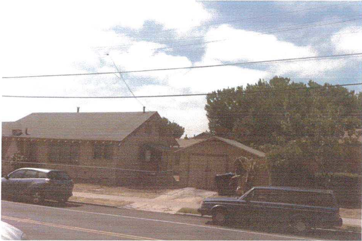
7. View looking South from site.
