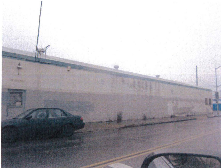
Looking at west elevation
