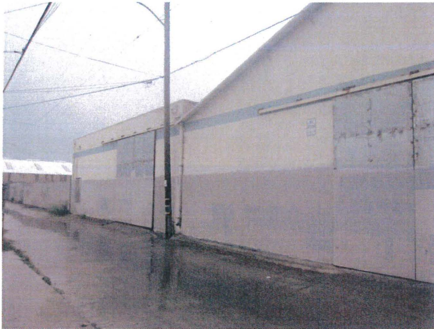
Looking at north elevation
