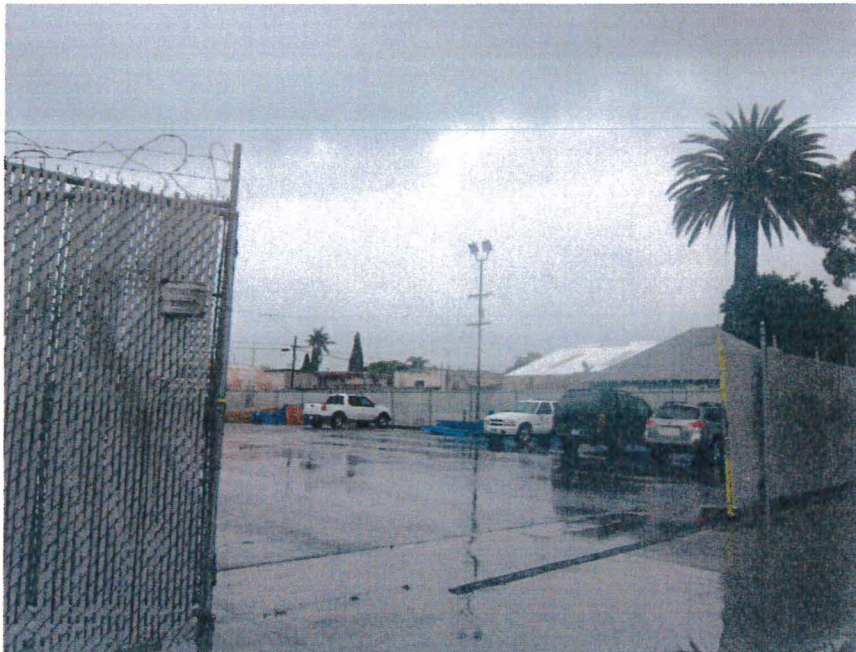
South view of the facility
