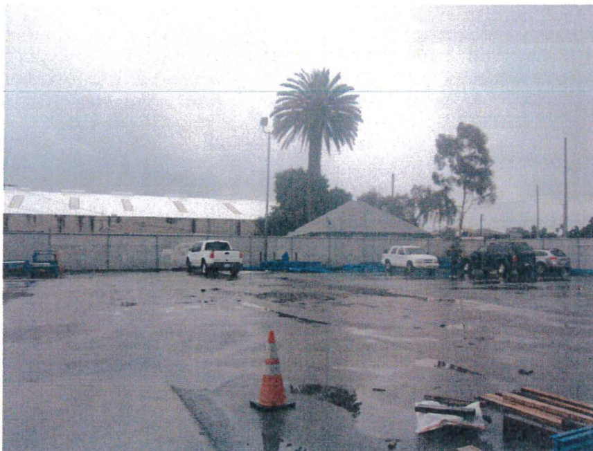
West view of the facility
