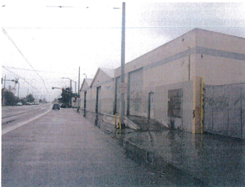
Looking at south elevation
