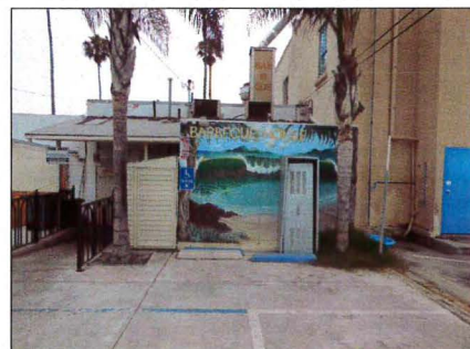
5025, 5027 Newport Avenue (South-Facing Rear Elevation)
