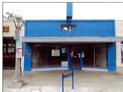
5029 Newport Avenue (North-Facing Elevation)
