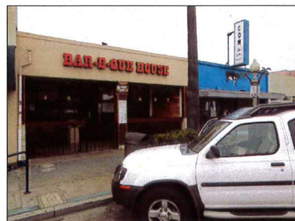
5025, 5027 Newport Avenue (North-Facing Elevation)
