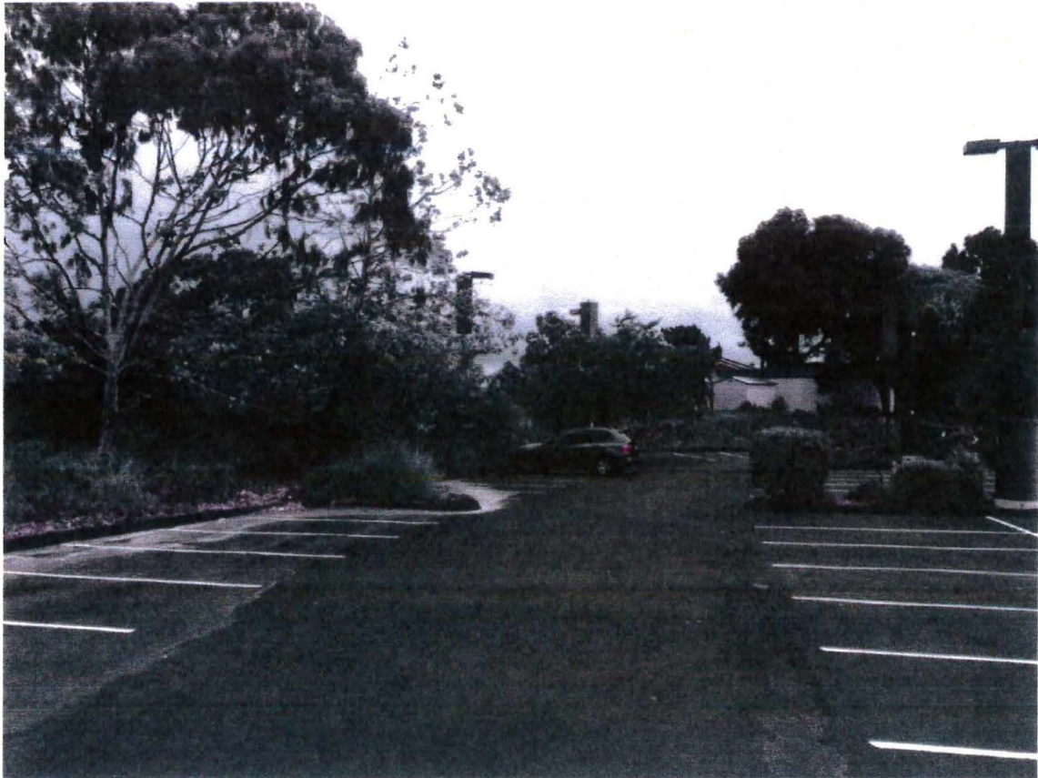
4. View of West Elevation of site.
