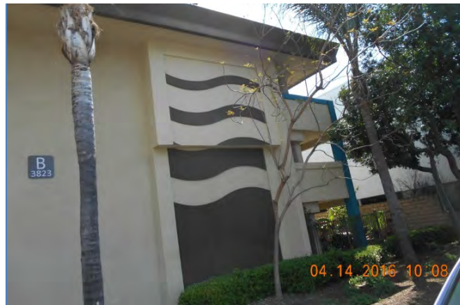
Figure 15: Although façade-mounted boxes are not preferred, this is still an excellent example of integration.
