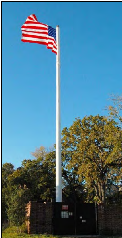
Figure 24: There are antennas in this flagpole.
