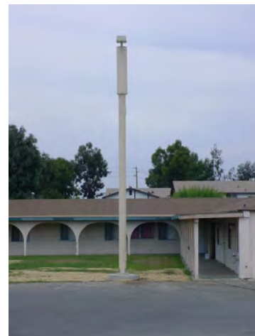
Figure 25: A parking lot light with an antenna shroud that complements the pole.
