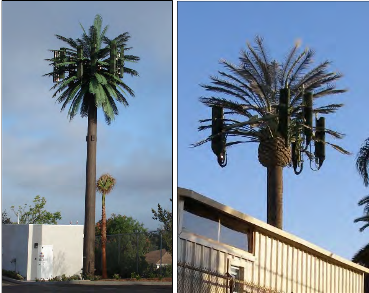
Figure 32: Faux palms do not provide the level of concealment required by the Wireless Ordinance - they are monopoles with fronds!
