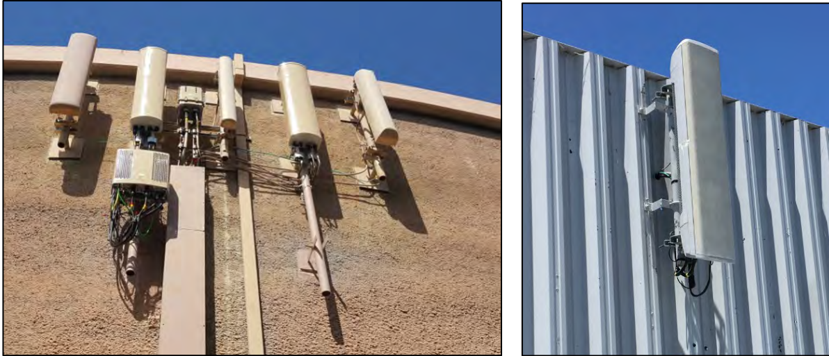
Figure 34: Unconcealed facilities like these do not meet the requirements of the Wireless Ordinance.
