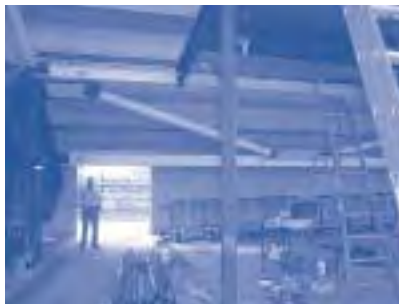
Petco Park submitted an appeal requesting omission of spray applied fire proofing.
