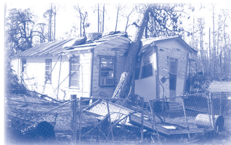
One of many structures that were uprooted by flood force and damaged by falling objects.
