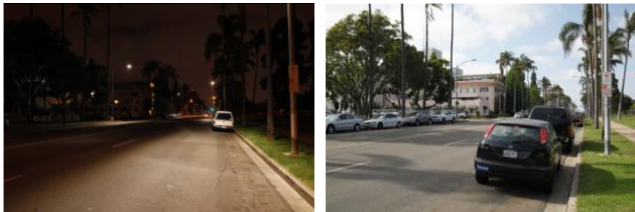
Figure 14: Nighttime and Daytime Photos of Test Area 4
