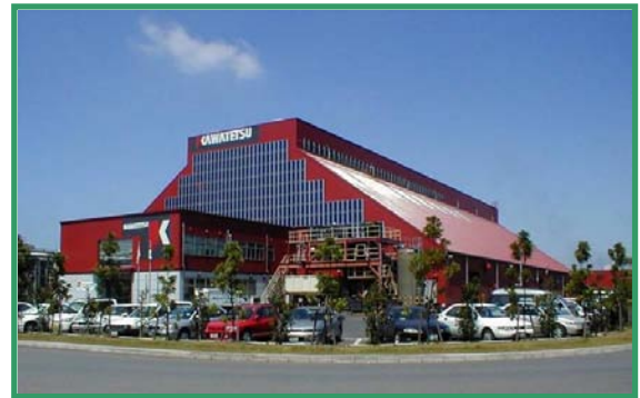
Thermoselect Facility Chiba, Japan
