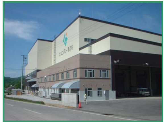
Plasma Gasification Facility Utashinai, Japan
