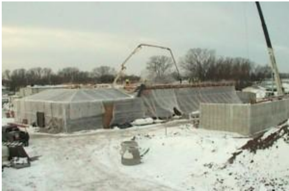
FIGURE 3-6 RECENT CONSTRUCTION PHOTO FROM BIOFERM™ (UNIVERSITY OF WISCONSIN – OSHKOSH)
