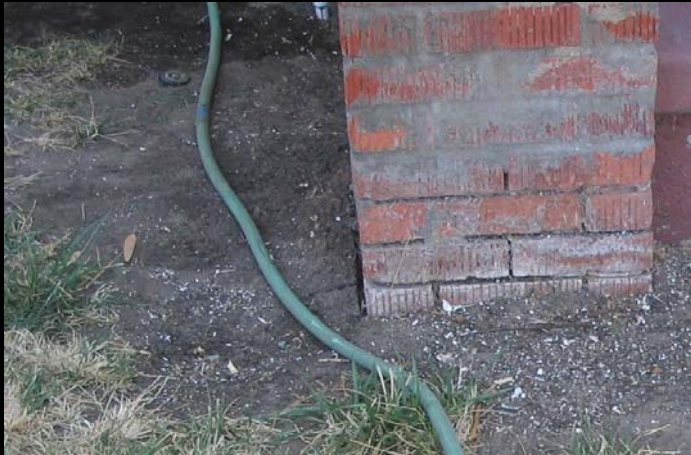
Paint Chips on Ground
