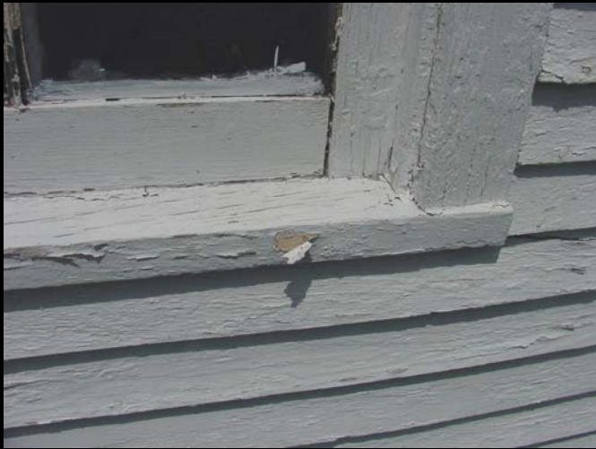
Exterior siding, window components
