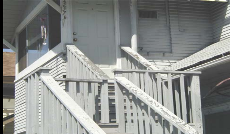
Deteriorated Stair Rails
