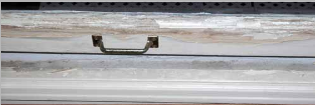
Deteriorated paint on bedroom window of a pre-1950 home
