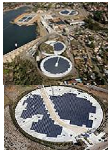
Photovoltaic system at Alvarado Water Treatment Plant
