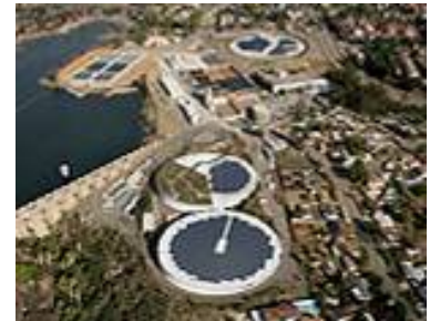
Photovoltaic system at Alvarado Water Treatment Plant
