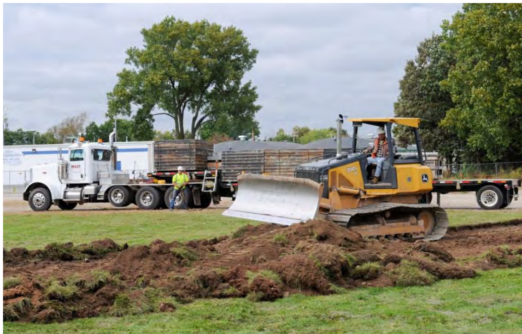
FIGURE 3-5 START OF CONSTRUCTION OF BIOFERM™ FACILITY (UNIVERSITY OF WISCONSIN – OSHKOSH)
