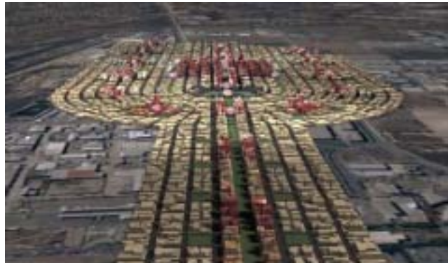
Figure 19: Aerial Approach to IBZ Central Business District
