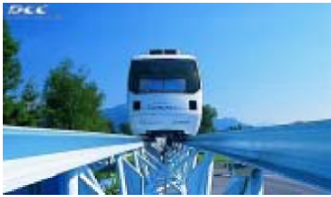
Figure 11: Tier 4 - Elevated Feeder Line
