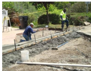
Storm Drain Maintenance
