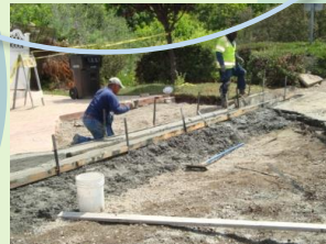
Storm Drain Maintenance
