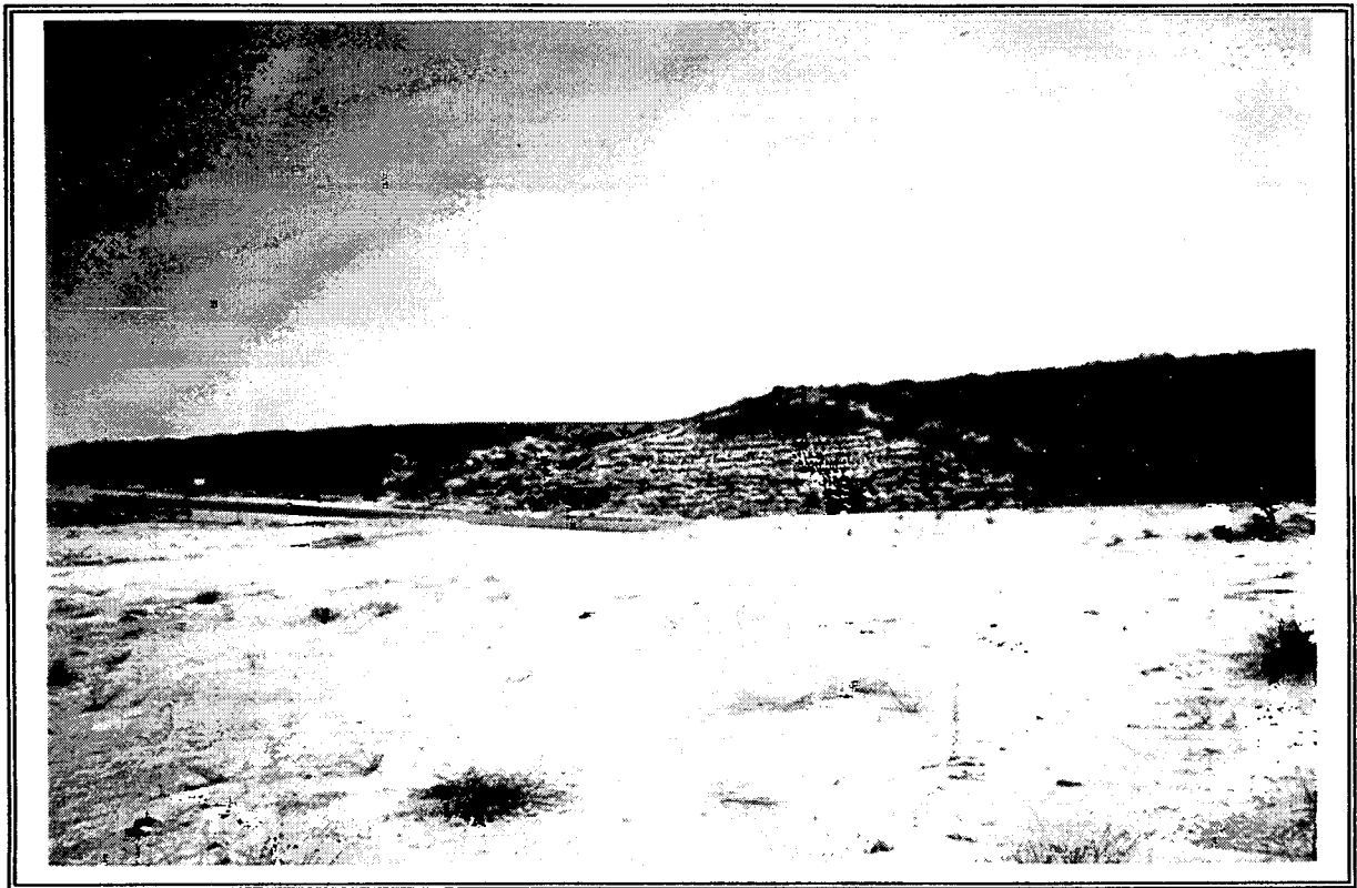
Pipefitters looking east across Camino Santa Fe (Pardee property in foreground)
