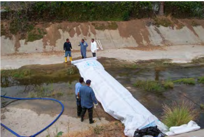
Inflated portable dam extended across storm channel, effectively blocking flow of water (storm water run-off in this case).
