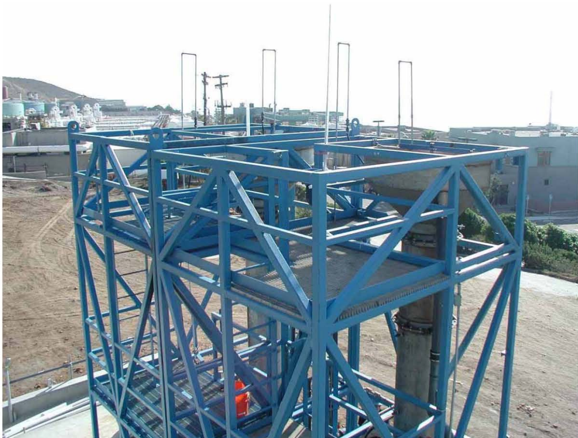
Picture 2. Biofor details. Top. Top structure showing media. Bottom. Top of columns, with Biofor C on the left.
