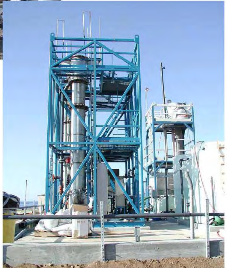
Picture 1. Pilot Plants. Top – Looking south, Biostyr on the left, Biofor C and N to the right and in the back. Bottom. Looking north, Biofor N on the left, Biofor C behind (not visible), and Biostyr to the right. Long pipes in the air are siphon breakers.
