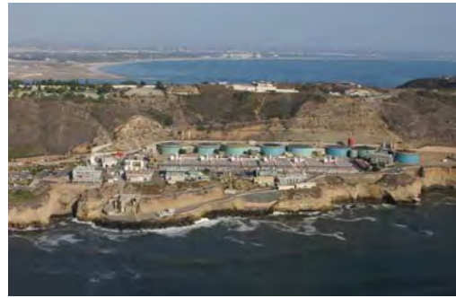
Figure 1.1. The Point Loma Wastewater Treatment Plant Can Treat up to an Average of 240 Million Gallons Per Day.
