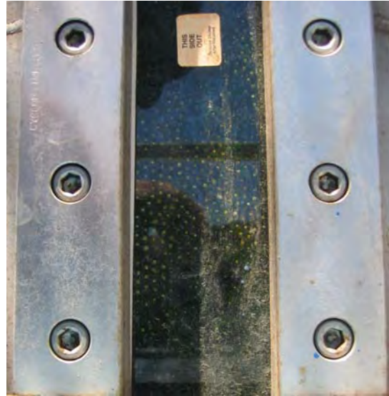
Figure 3.4. Photo of Media in Biostyr Column as Seen Through Observation Window
