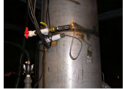
Figure 3.5. Photo of Pressure Transducer Mounted on BAF Column
