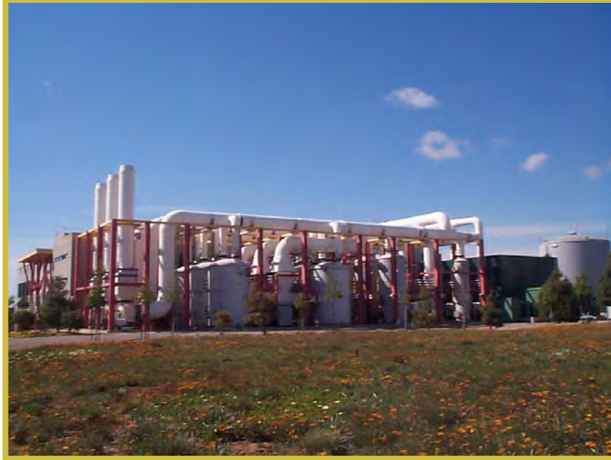
ODOR CONTROL FACILITY
