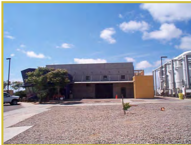
WASTEWATER PUMP STATION
