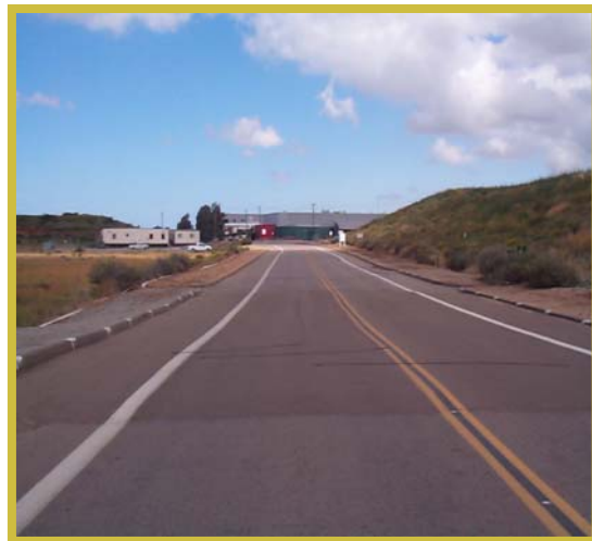
MBC ACCESS ROAD
