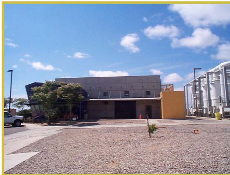
WASTEWATER PUMP STATION
