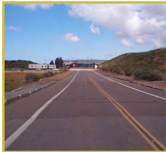
MBC ACCESS ROAD
