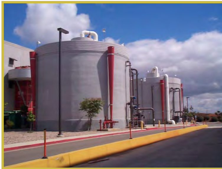
RAW SOLIDS RECEIVING TANKS
