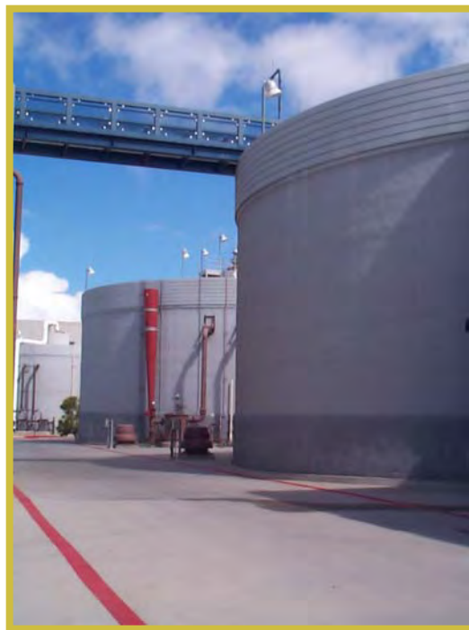
DIGESTED BIOSOLIDS STORAGE TANKS
