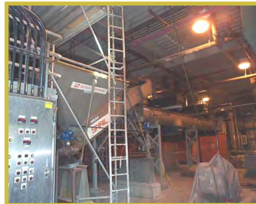
GRIT DEWATERING UNIT AND SCREW CONVEYOR
