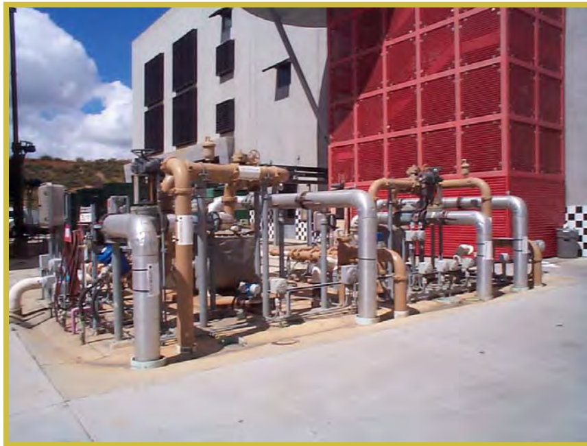
TOP OF BLENDING TANKS
