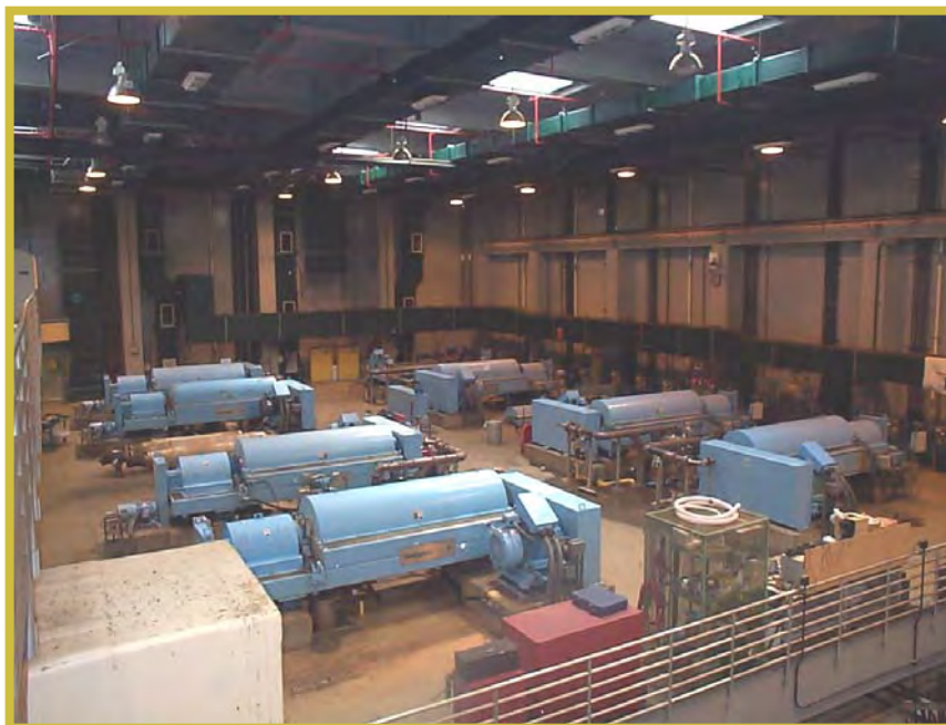
DEWATERING CENTRIFUGES
