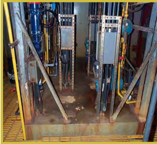
FERRIC CHLORIDE FEED AND TRANSFER (RIGHT) PUMPS
