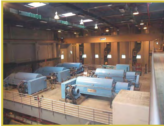
THICKENING CENTRIFUGES
