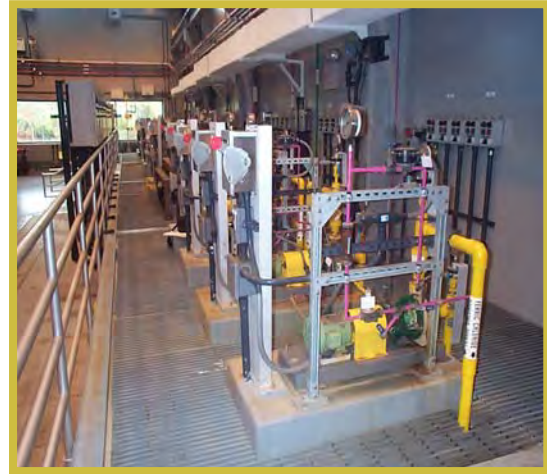
FERRIC CHLORIDE FEED AND TRANSFER (RIGHT) PUMPS
