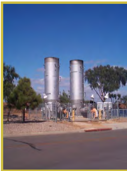
WASTE BIOGAS FLARES
