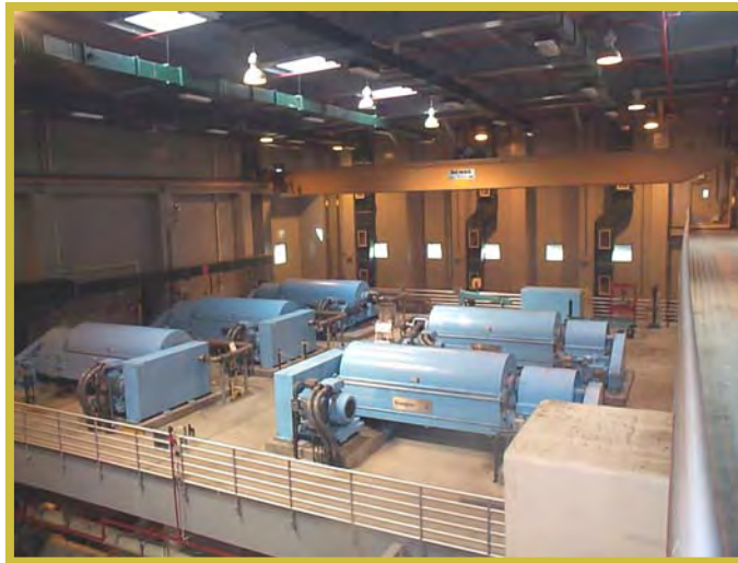
THICKENING CENTRIFUGES
