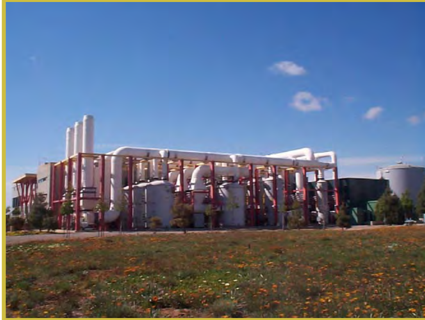
ODOR CONTROL FACILITY
