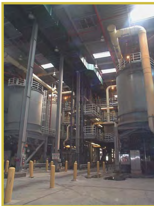
DEWATERED BIOSOLIDS STORAGE BINS AND TRUCK LOADOUT STATIONS
