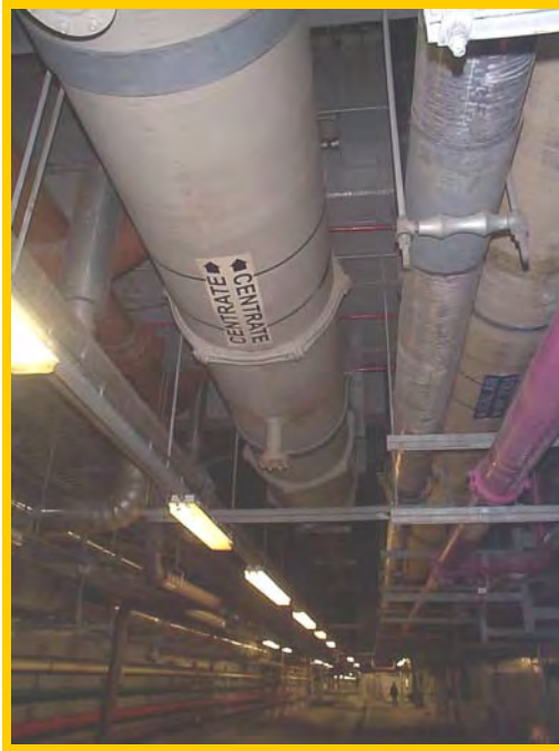
CENTRATE PIPE HEADER IN THE PIPE GALLERY
