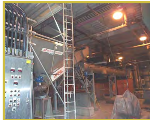
GRIT DEWATERING UNIT AND SCREW CONVEYOR
