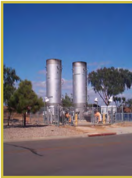
WASTE BIOGAS FLARES
