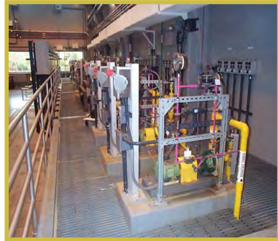
FERRIC CHLORIDE FEED AND TRANSFER (RIGHT) PUMPS
