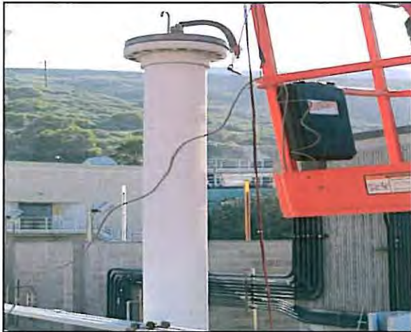
Photo 3: Transducer is Inserted Into Static Water Well for Testing
