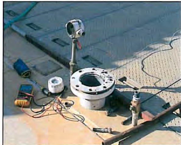
Photo 2: Flume Access After Transducer Was Removed
