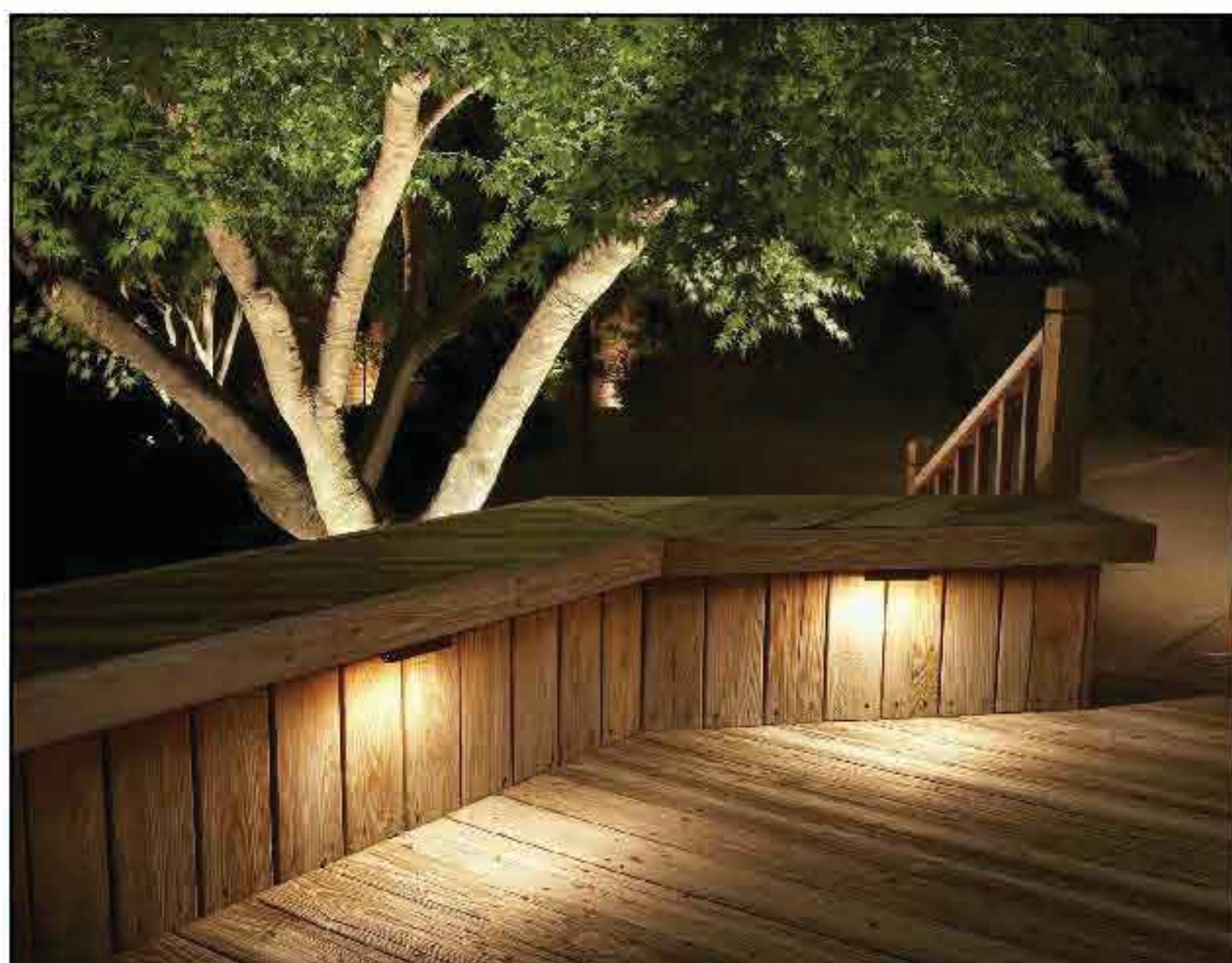
WALL NICHE LIGHTS AND VEGETATION UPLIGHTS
