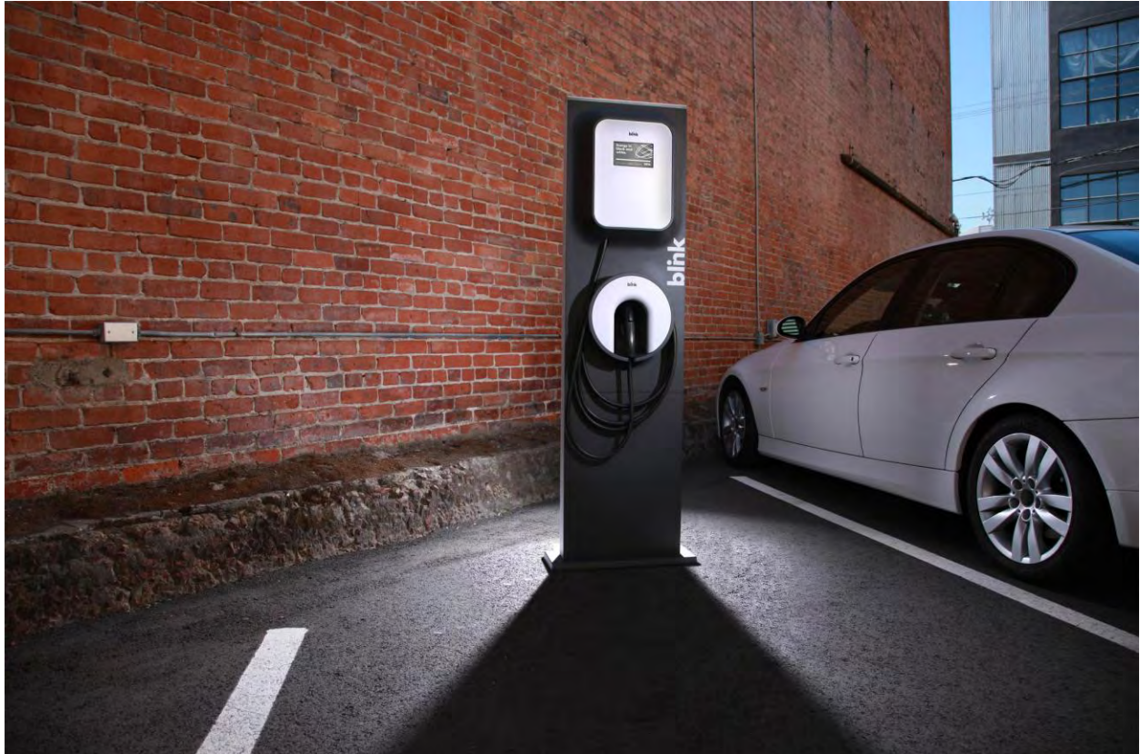
Below – EV Charging Station in context.
