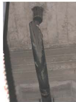
Photo of Bent 6 - interior broken down drain before repairs were made.
