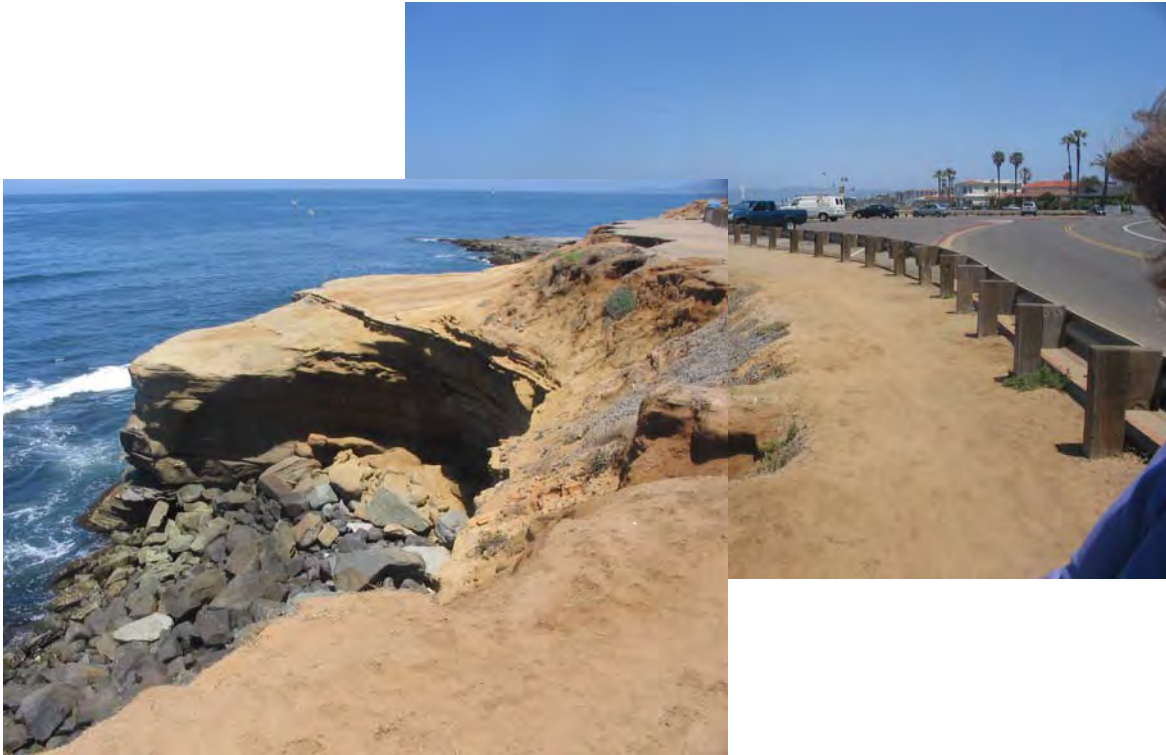
PH13/14: riprap placed by the Corps in 84/86. Parking lot at Osprey.
