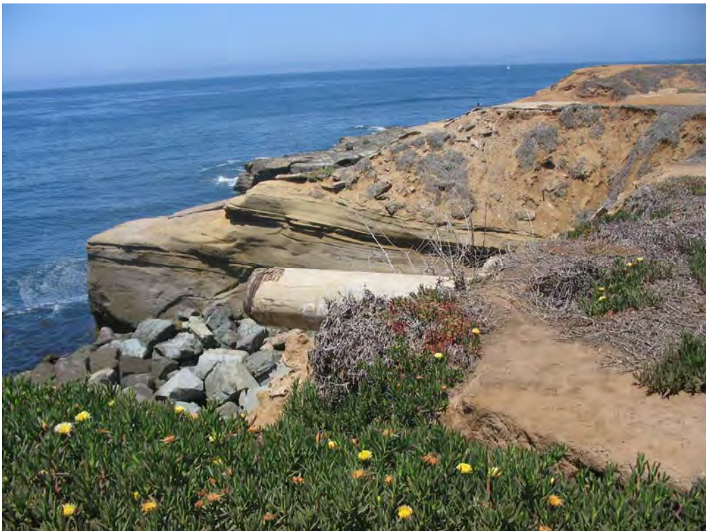
PH20: Osprey drain pipe filled below with rip-rap. Drain pipe to be removed with new plan.
