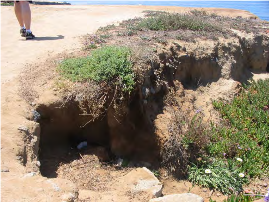
PH 12: There is un-natural fill material placed on the top of the bluffs from the Corps during the same 1984?
