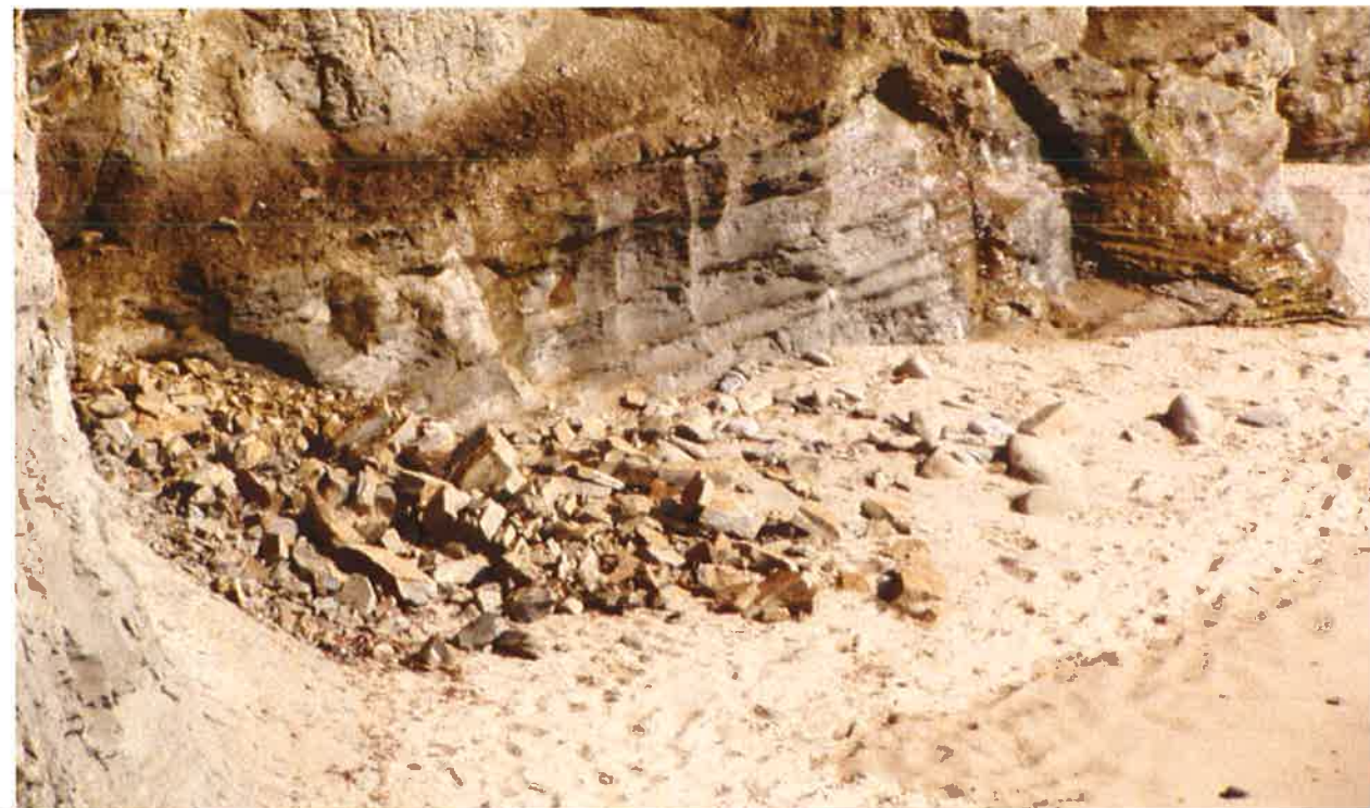
Figure 37. Northern end of Garbage Beach where runoff from the northwest corner of the Lower Parking Lot discharges over the cliff. Cliff block falls in this area pose a clear danger to beach users below as illustrated by these two photos taken 2 weeks apart.
