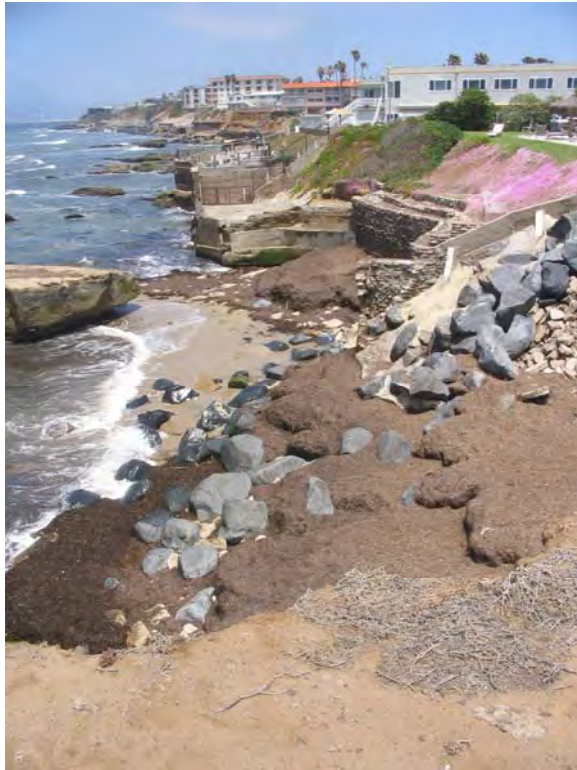
PH29: This shows 'unnatural' erosion caused by failing and settling rubble. Dedi would like to see a set of terraces/stairs at this point to view the entrance of the park.
