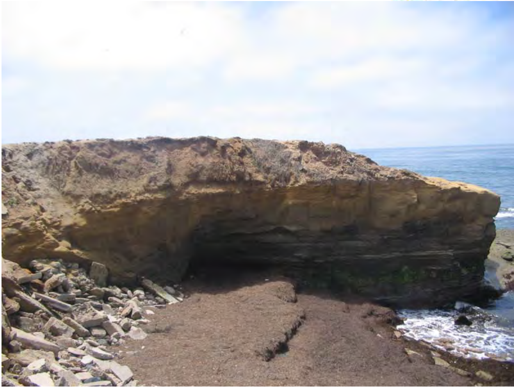
PH32: Construction rubble over bluff.
