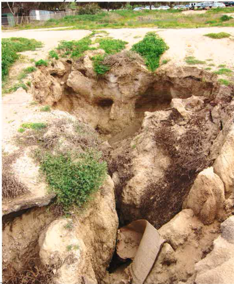
Figure 33. Bluff erosion caused mainly by runoff from the southwest corner of the Lower Parking Lot. This erosion and that shown in the previous figures could be eliminated by putting curbs and berms in the southwest portion of the Lower Parking Lot.
