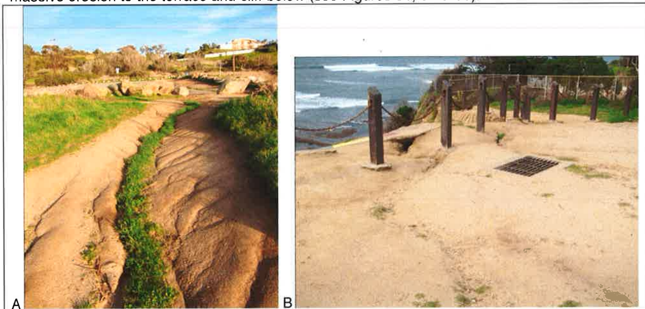
Figure 29A & B. Runoff gully from the southwest corner of the Lower Parking Lot leading an inlet on the bluff above the Gunite swale. The inlet and swale are higher than the erosion gullies cut around them, therefore the runoff continues to bypass the drainage system and is undermining the Gunite drainage swale. These maintenance problems should be addressed before the system is irreparably damaged.
