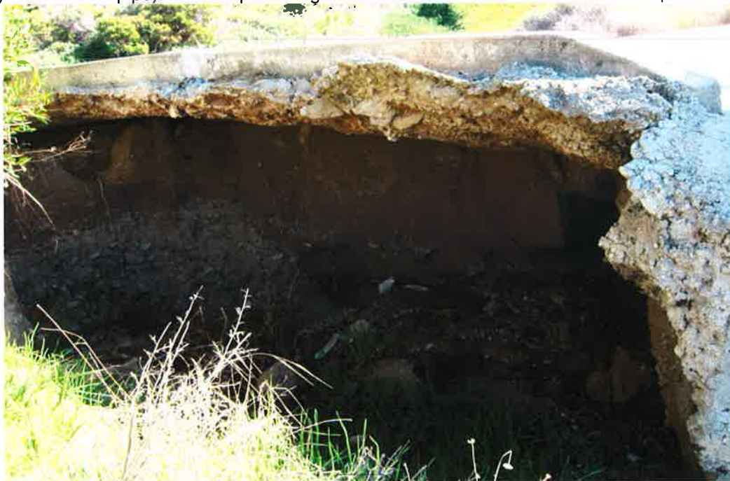
Figure 25B. Close up of the undermining of the Loop Road Arizona Crossing. Most of the water causing this damage is from the 24" drain.
