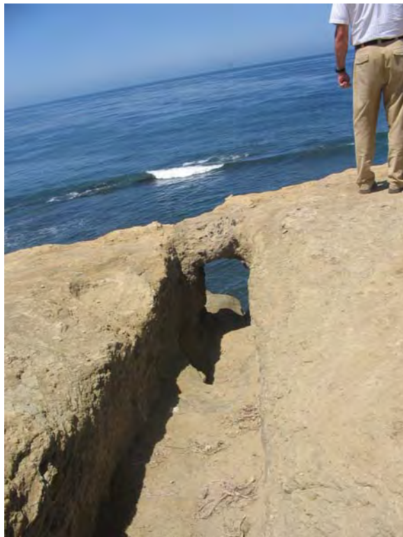
PH9: Remnants from a 1915 wooden drainage structure.
