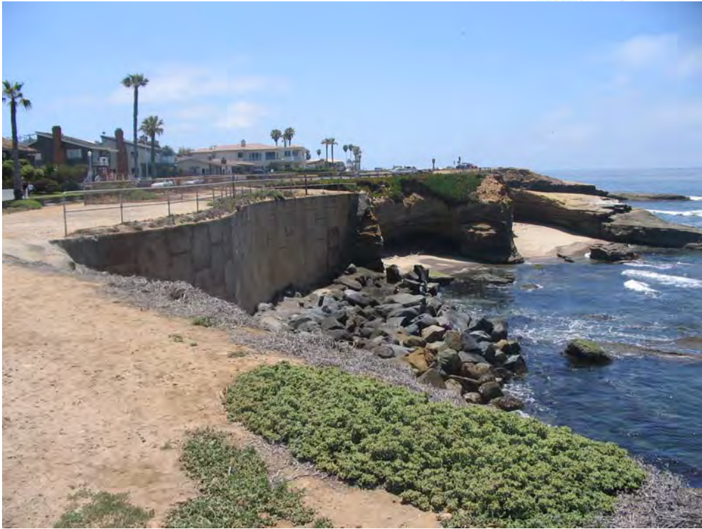
PH27: Dedi recommended 'stair-stepping' the bluff down to restore this area (opposed to hard vertical wall) (Looking back toward area of photo 26. we were out on the seaward point looking landward)
