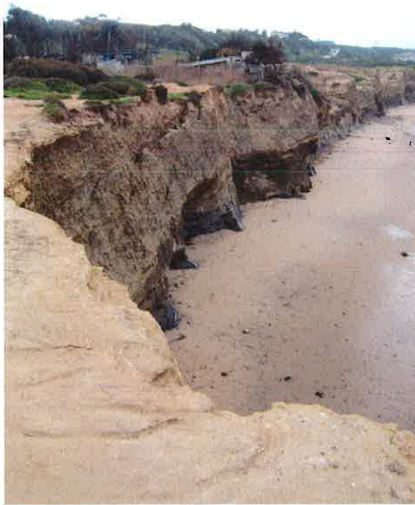
Figure 36. Runoff discharge from the NW corner of the Lower Parking Lot occurs all along this cliff above Garbage Beach. This dangerous cliff loss could be eliminated by diverting as much runoff as possible in the northern portion of the parking lot to the drain inlet in the southwest corner. Wattles and trail bars in the Eucalyptus grove should be used to build soil, and slow and spread the runoff so it isn't concentrated in one watercourse as it is now.
