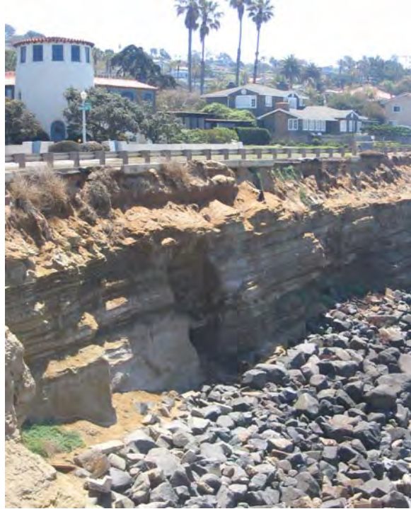
PH6 &7: Bluff Top erosion. 5 years ago this was very small and now it is large and you cant walk over it anymore. 5 years to create this hole.
