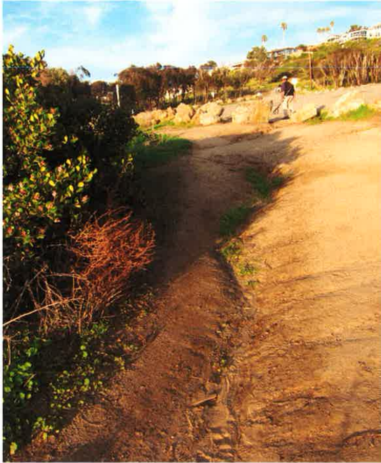
Figure 30. Runoff from the southwest corner of the Lower Parking Lot, that has bypassed the storm drain, mostly follows this trail that runs southwest. This trail is planned as ADA. If the runoff is not abated, a raised walkway will need to be installed to provide an adequate surface for an accessible path.
