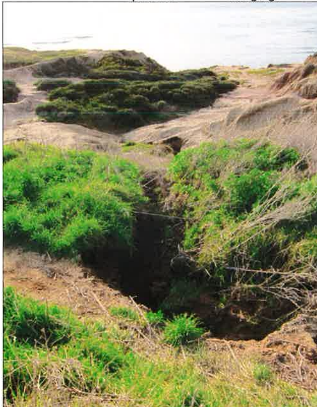
Figure 15. Southern part of the new erosion gully formed by runoff from the 18" drain where it runs into the Badlands. This runoff flows into Culvert Canyon and into the nearshore waters.
