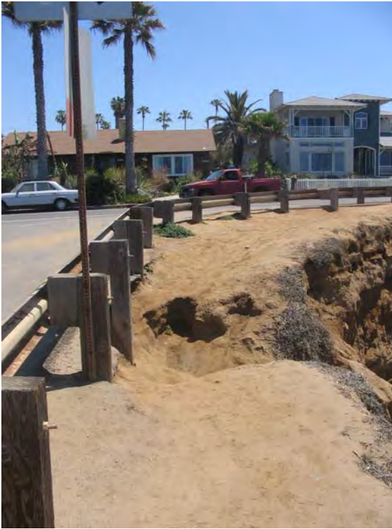
PH6 &7: Bluff Top erosion. 5 years ago this was very small and now it is large and you cant walk over it anymore. 5 years to create this hole.
