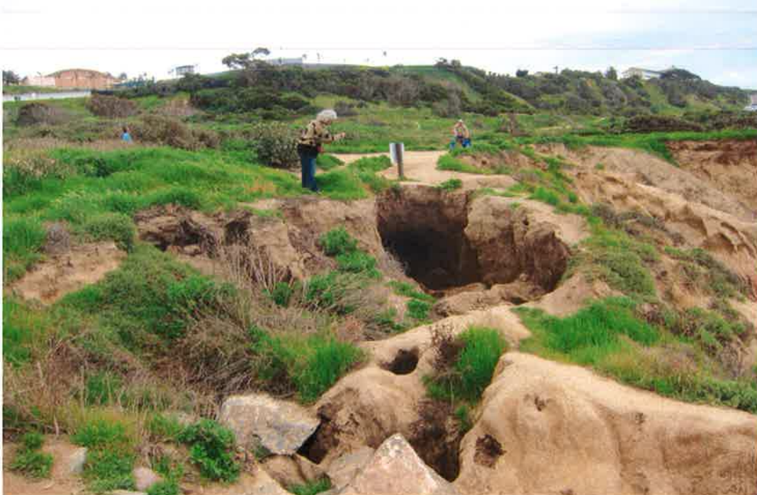
Figure 31. Bluff erosion caused mainly by runoff from the southwest corner of the Lower Parking Lot.
