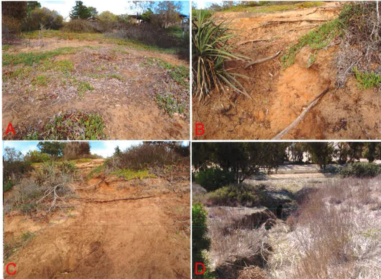
Figure 27. Area of Park where pedestrian traffic appears to have denuded the hillside (see A, B and C). Without a good cover of native plants, rainfall doesn't sink into the ground resulting in runoff generation that is causing erosion down slope, just before the runoff enters the Lower Parking Lot (see D).
