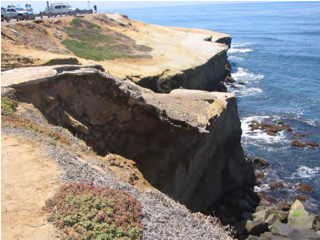
PH21/22: Another “failed” attempt to control runoff erosion of bluff, by pouring a concrete slab over the top of the point. These things need to be removed.
