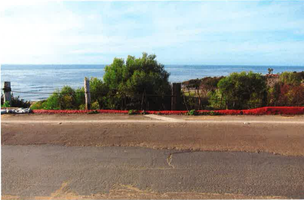
Figure 9. The curb height changes from 6" to 3" allowing storm water to run off between the two Acacia trees by the unpainted wood post, as well as, where the curb is missing, down slope from the sand bags.
