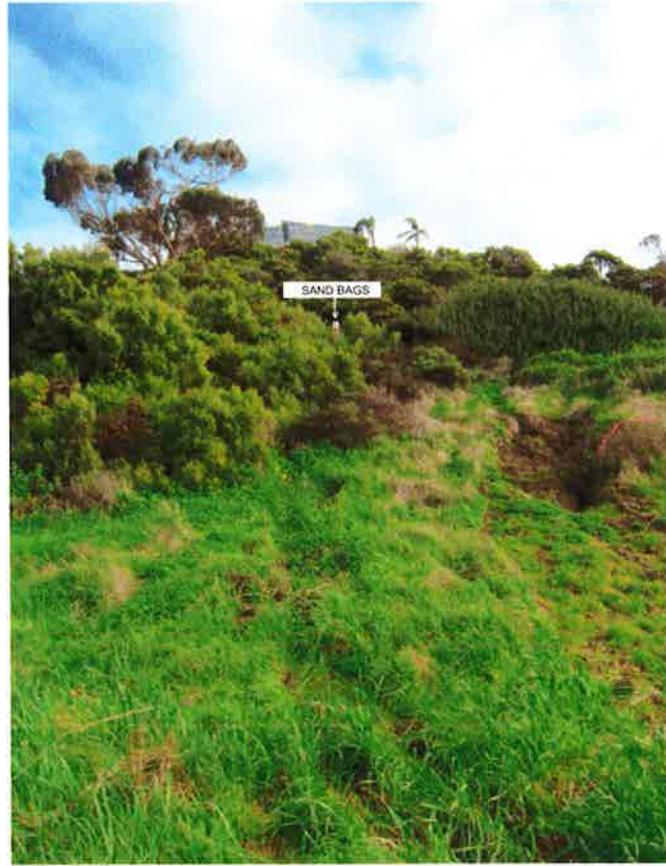
Figure 11A. This runoff course, due to the 18" pipe, is slightly further down the Loop Road than is the one shown in Figure 10. The runoff caused the "trail" and the slump and erosion to the right.
