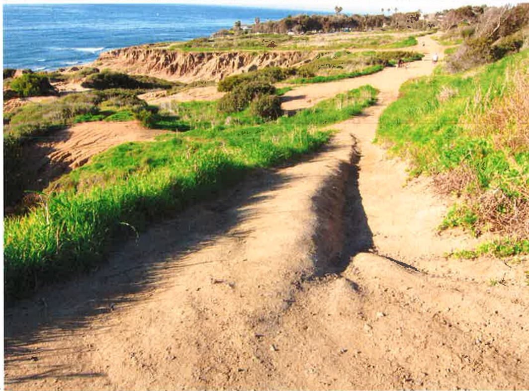
Figure 22A & 22B. Low curbs transition to 6" high curbs where the ramp from the sludge line trail joins the Loop Road (Figure 22A). The low curbs enable road runoff, made up in large part by discharges from the 24" pipe, to flow down the transition trail (Figure 22B) and into Culvert Canyon where it contributes to
