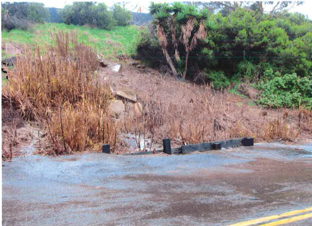
Figure 6. Runoff and erosion features associated with the 18" PLNU drainage pipe that discharges onto the Loop Road at the marked location. The large red dots show the location of features, and the small dots and streamlines show where evidence of watercourses transporting runoff that ponds on the Loop Road due to discharges from the 18" pipe can be seen after major rainfall events.
