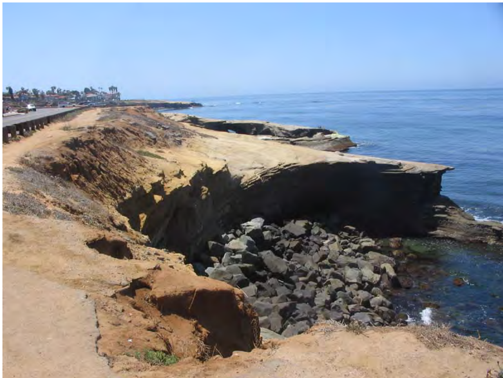
PH15: (From parking lot at Osprey). Dedi used to walk across these two points as a kid, it used to be straight across. It has since eroded into a small cove area and rip-rap has been placed at foot of bluff in cove.
