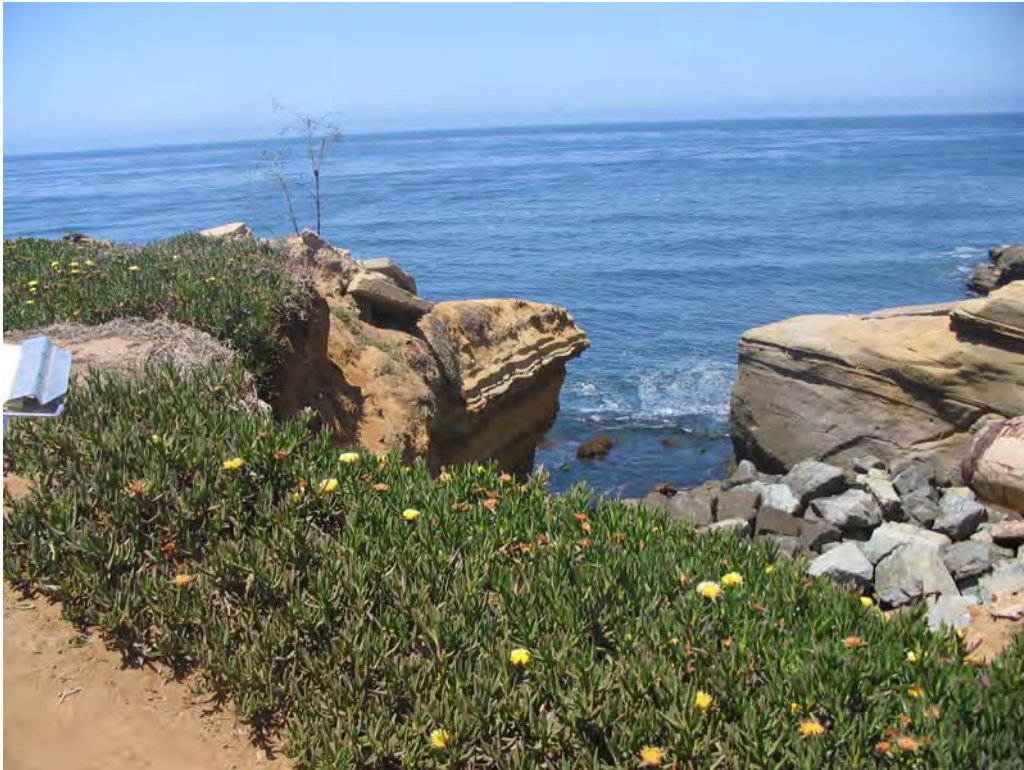
PH19: at Osprey street: rubble at the end of the point. Needs to be removed. Does this increase erosion from the added weight of riprap/rubble on top of the bluff?
