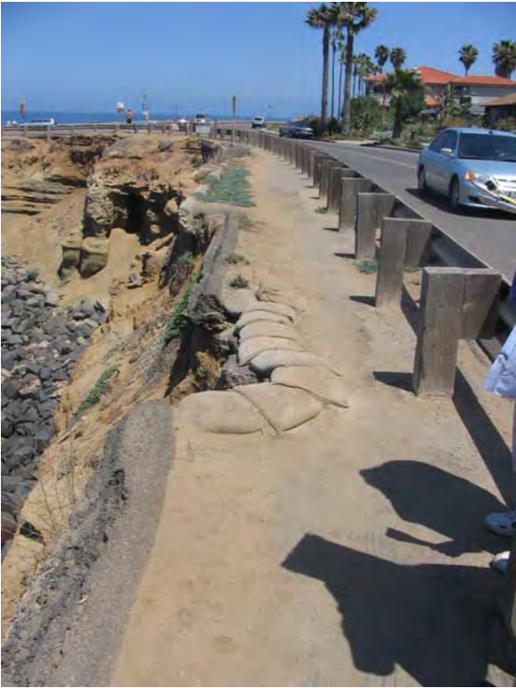
PH1: Sandbags at the end of Fronde Street to prevent runoff over cliffs
