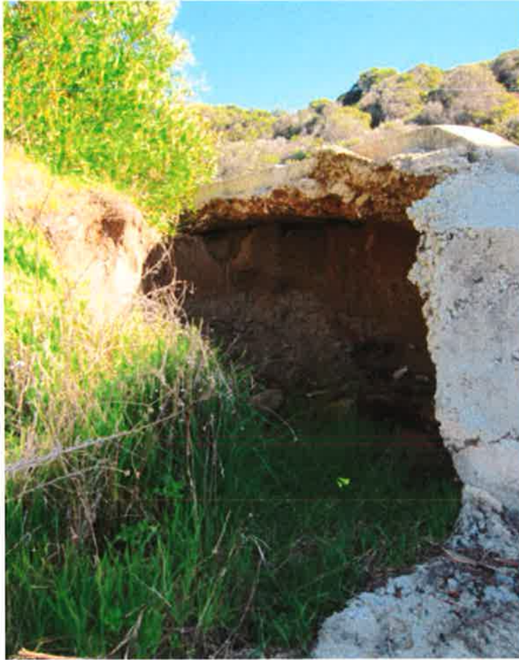
Figure 25A. Undermining of the Loop Road Arizona Crossing by runoff that flows over the western curb (primarily from the 24" pipe). An adequate height curb could eliminate this maintenance problem.
