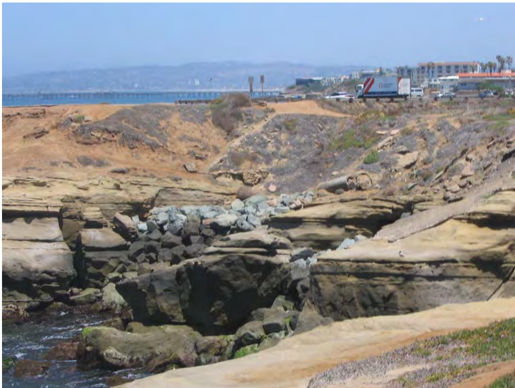
PH17/18: Fill on cliff face the end of Osprey.
