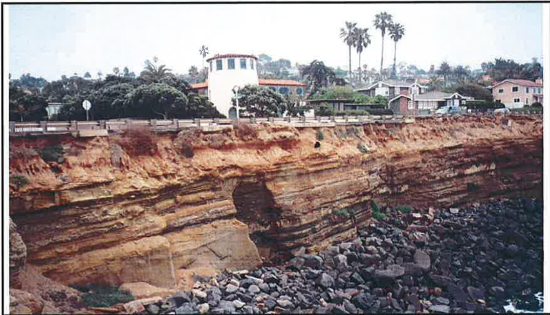
Figure 4C: Bluff face in front of Froude Street intersection. Moderately sloping and eroding terrace deposits of Bay Point Formation overlying sedimentary rock of Point Loma Formation with rip-rap protecting base of bedrock.
