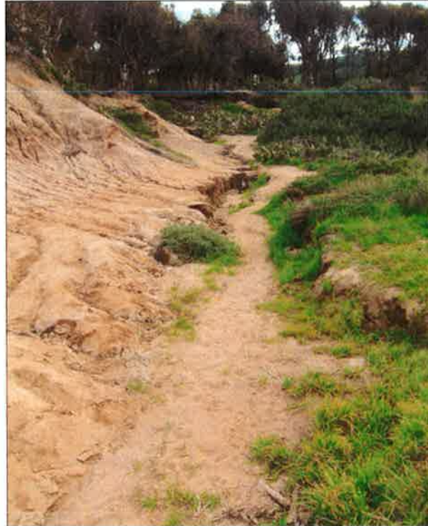
Figure 35. Erosion gully that receives runoff from the northwest corner of the Lower Parking Lot after it has run through the Eucalyptus grove (Figure 32).
