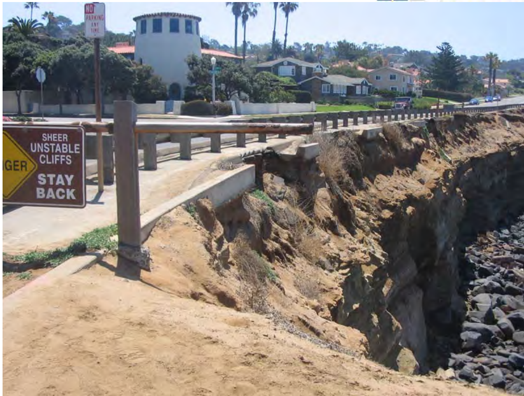
PH4: Bluff Failure caused by 2 caves joining on both sides of bluff protrusion and water impact through these formations.
