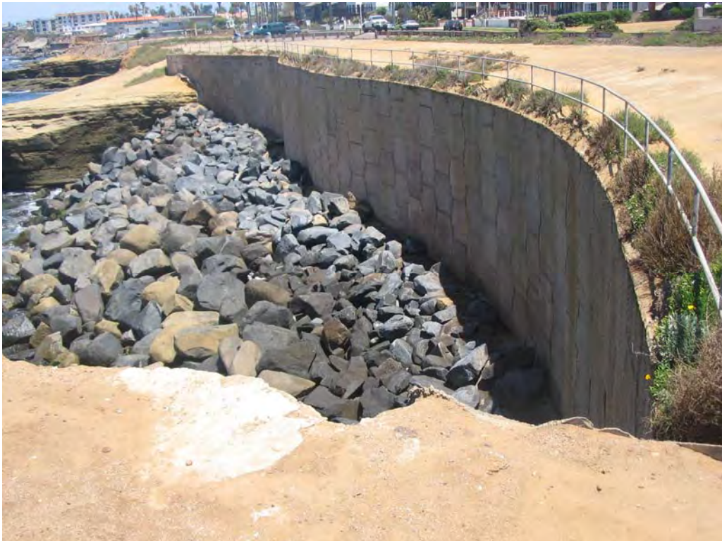
PH24: USACE sea wall/riprap. There was a cove behind it that extended close to the road. The Corps built the wall farther seaward and filled behind it. The fill appears to be quarry rock and dirt. Dedi would prefer to see this are be used as a parking area, since it is 'man made' and it would be hard to restore this are to natural conditions. Natural vegetation would have a hard time growing over the fill material.
