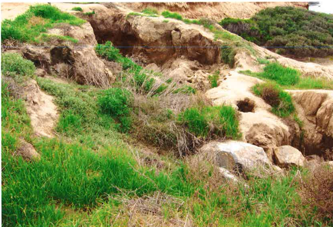
Figure 32. Bluff erosion caused mainly by runoff from the southwest corner of the Lower Parking Lot.
