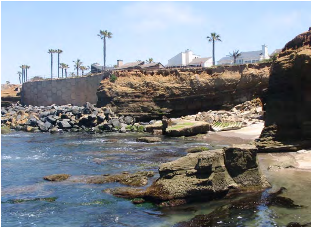
Photo 4 –Northern seawall showing location where a new seawall could be implemented, Site 9.
