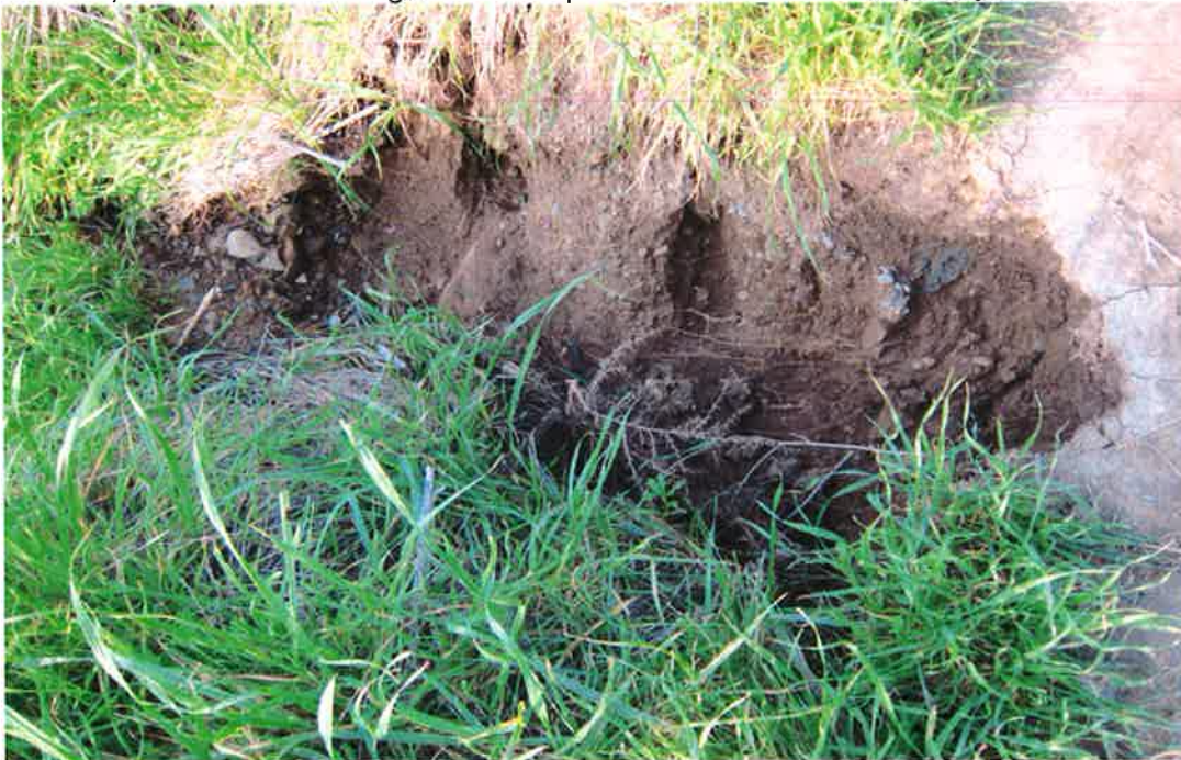
Figure 12B. Close up of erosion washing out the path. 6" curbs along the Loop Road could easily eliminate the runoff causing this washout and allow this trail to be part of the permanent trail system.
