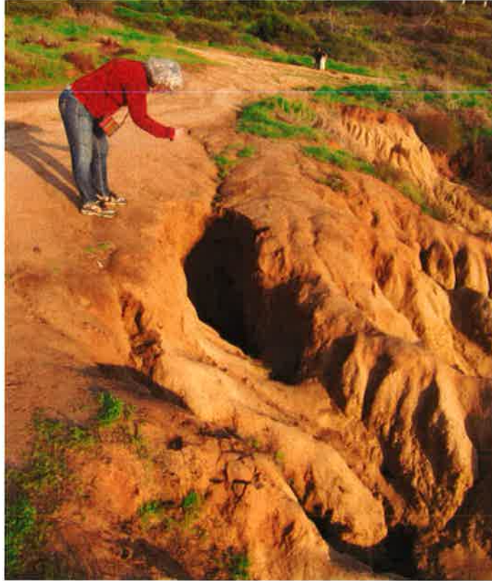
Figure 16. Additional erosion caused by discharges from the 18" pipe along the northern edge of the Badlands. 6" curbs on the Loop Road could easily control this erosion.
