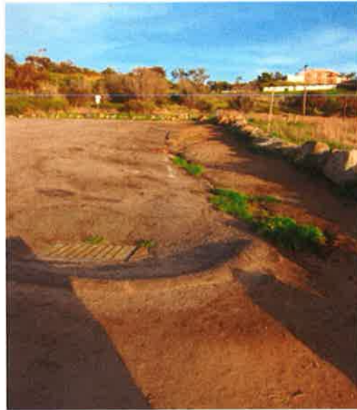
Figure 28. The south side of the Lower Parking Lot, showing both the storm drain inlet and an erosion gully to the south of the storm drain inlet. Clearly, runoff from Drainage Basin I flows along the south side of the lot, causing rill and gully erosion before it discharges over the cliff (Figure 24).
