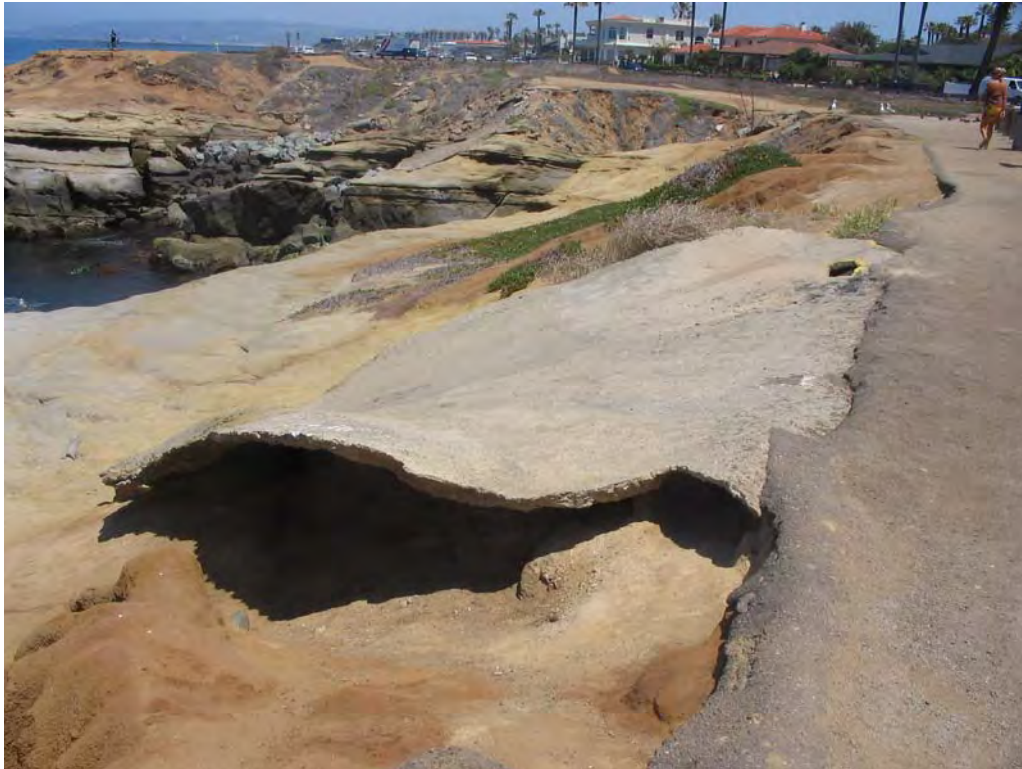
PH16: Concrete slab placed as a (failed) attempt to control run-off erosion (at Osprey). Flow was supposed to go over it, but as shown, it has scoured around it. Rodents live under these structures as they provide extra protection.
