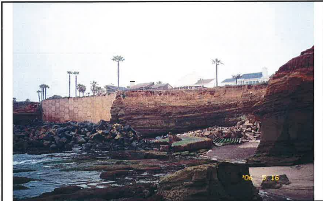
Figure 4B: MSE wall for bluff stabilization along with rip-rap at base near Adair Street. Terrace deposits of Bay Point Formation seen overlying Point Loma Formation.
