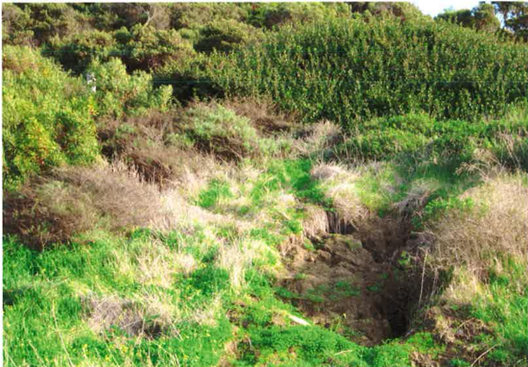
Figure 11B. Close-up of the erosion/mass wasting/mud hole due to runoff from the Loop Road. Those who use this trail to access surfing areas on an almost daily basis did not observe this damage to the Park prior to the December 2010 storm.
