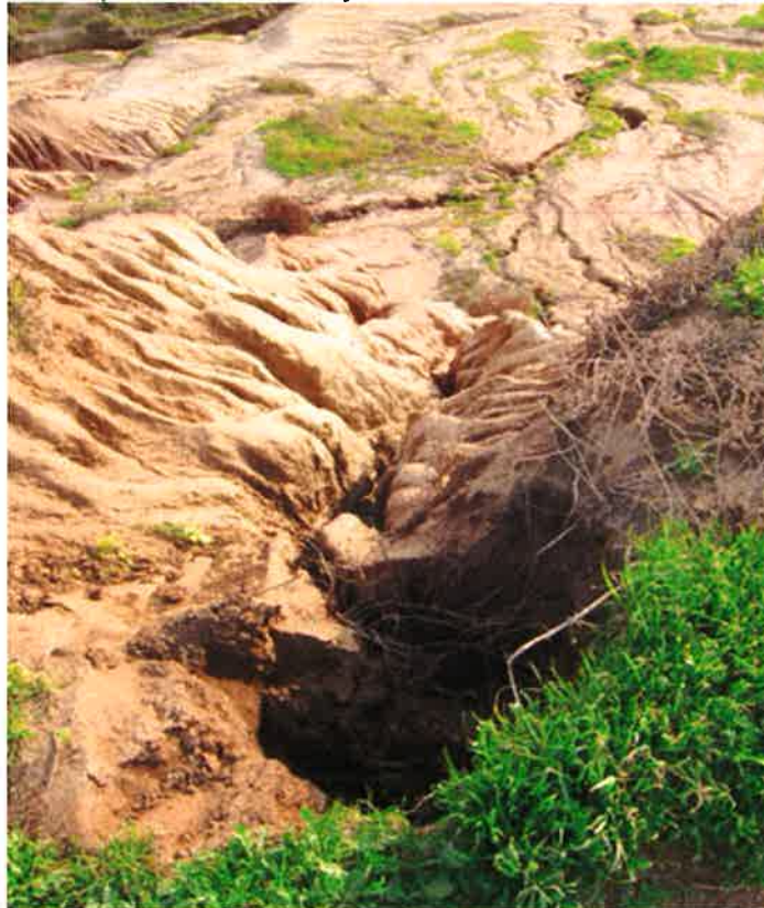
Figure 17. One of many sinkholes next to the trail in the Badlands that pose a clear danger to people and pets, because they are over 10" in depth. These are caused by runoff from the 18" pipe.
