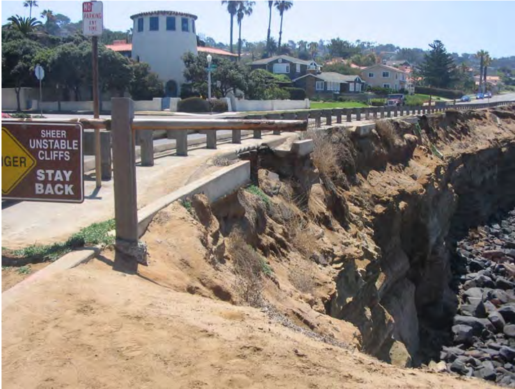
Photo 8 – Top of Bluffs, showing damage to curb, Site 7.
