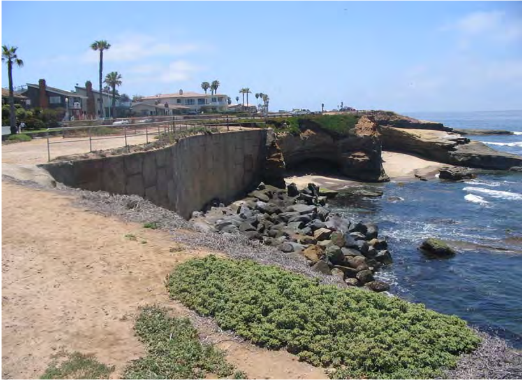
Photo 3 –Southern seawall, just north of Spaulding Point, Site 9.
