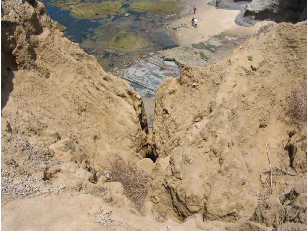
Top of “V” that is shown in previous pictures from Garbage beach. This has eroded significantly over the last 5 years.
