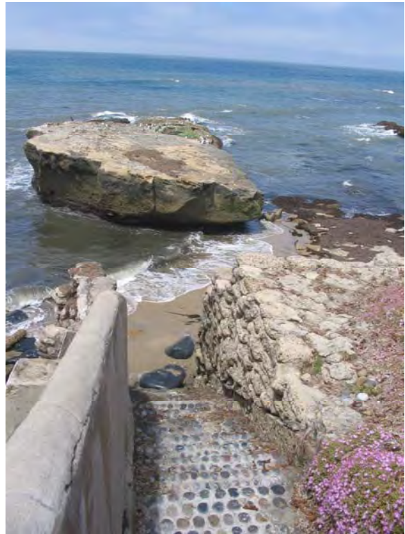
PH30/31: historical steps (1915), ended on sand to walk across to large rock. Now there is a big drop down and no sand along this reach. (Man-made 'swimming' hole in rock)
