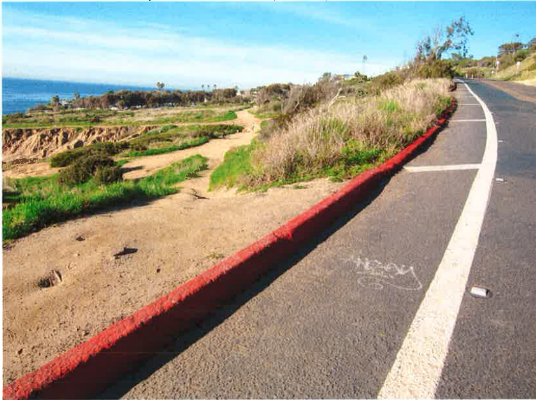
Figure 21. Erosion rills cause by runoff from the Loop Road, predominantly from the 24" pipe.
