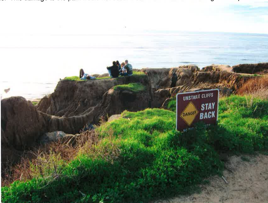
Figure 19. Runoff from both the 18" pipe and the Upper Parking Lot are likely responsible for this massive loss of cliff.
