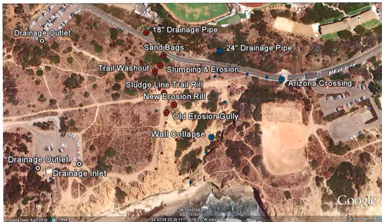
Figure 3. Areas in the Hillside Park where erosion and mass wasting problems can be corrected, by constructing curbs along the Western Loop Road. Features, both constructed and due to erosion, associated with discharge from the 18" drainage pipe are shown with red dots and those with the 24" drainage pipe with blue dots. The Lower Parking Lot's main features are shown in white.
