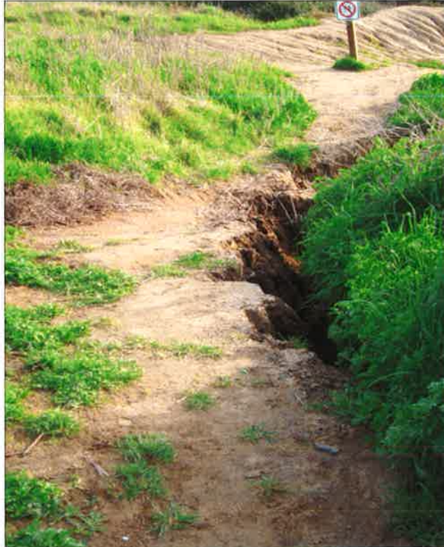
Figure 14. This new erosion gully from runoff from the 18" drain coming off the Western Loop Road was first noticed after the major December 2010 storm. The upper, southward running portions of this recently formed gully should be filled in and stabilized to prevent it from enlarging.
