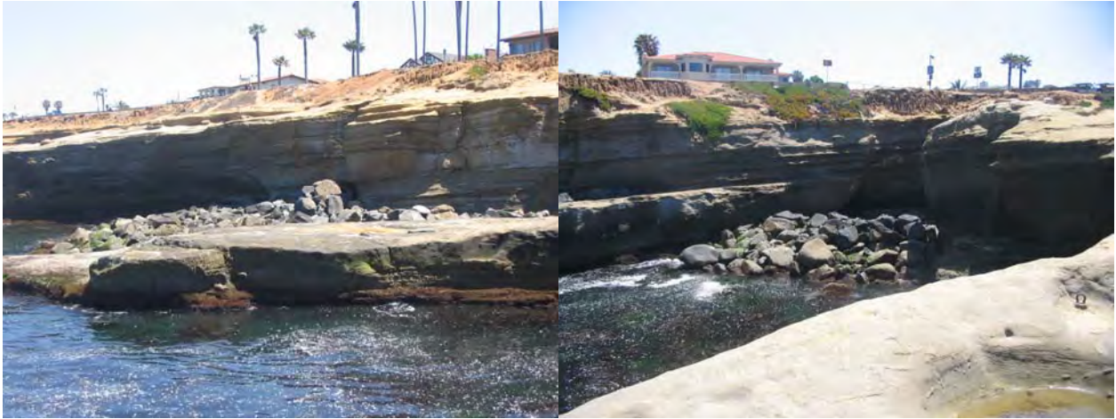
PH10/11: Riprap to fill coves. In 1984, the Corps filled in all the crevices and eroded areas along entire SCB stretch.
