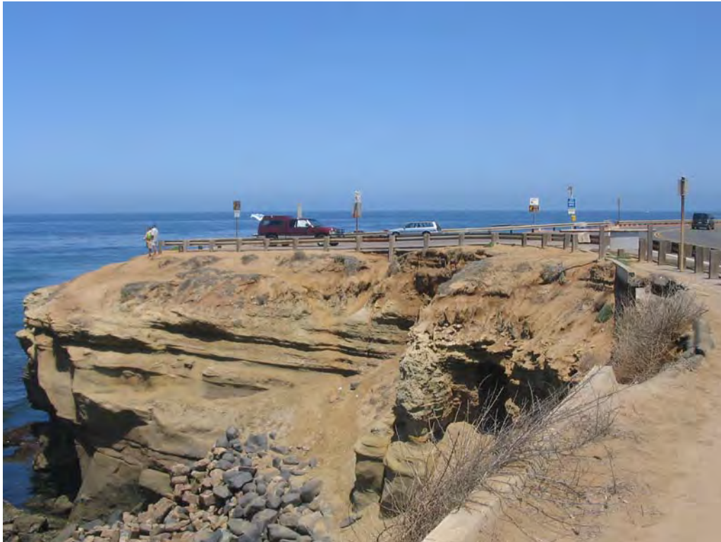
PH3: Parking at Froude Street slopes seaward; therefore all drainage runs over cliff. Concrete stairs used to exist to get to the cave and were replaced in the 1940s (these lasted 10-15 years). In 1915, near the corner of the parking, there was a little building there (this is where there was a lot of bluff erosion).
