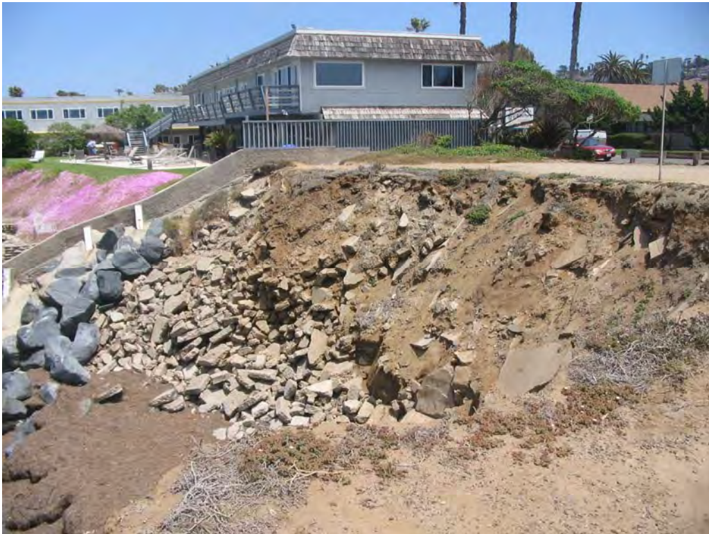
PH28: construction fill, concrete rubble. 1930 whole caved in and rubble fill was placed.
