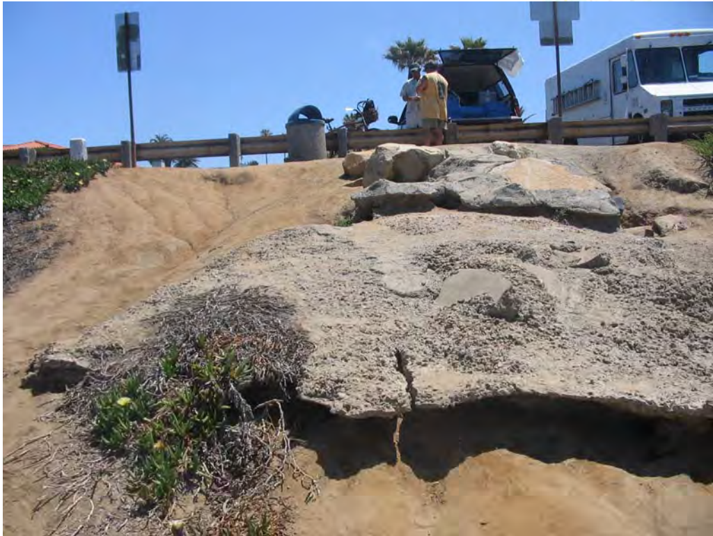
PH8: showing concrete and eroded gullies from rain run-off from the parking lot.
