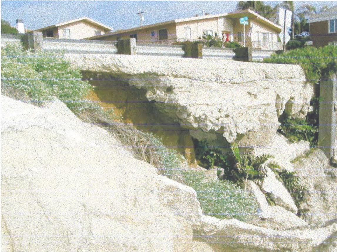
**Recommendations:** Rick Engineering recommends a major upgrade of the drainage system that discharges over the cliff at Location 9 that would include the replacement of four sections of pipe totaling 730 feet in length. This upgrade needs to be implemented in order to protect the cliffs from further erosion, and prevent Sunset Cliffs Boulevard from being undermined.
