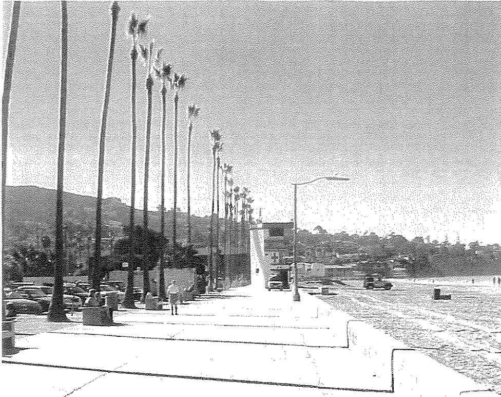
F) View of Existing Boardwalk Looking South & Existing Lifeguard Station
