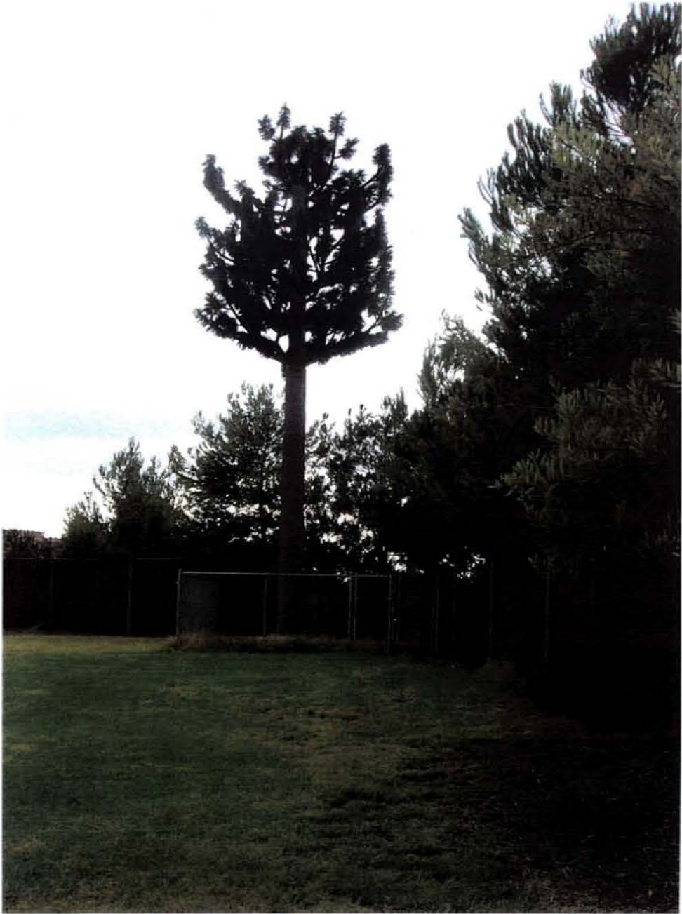
Existing Verizon monopine.
