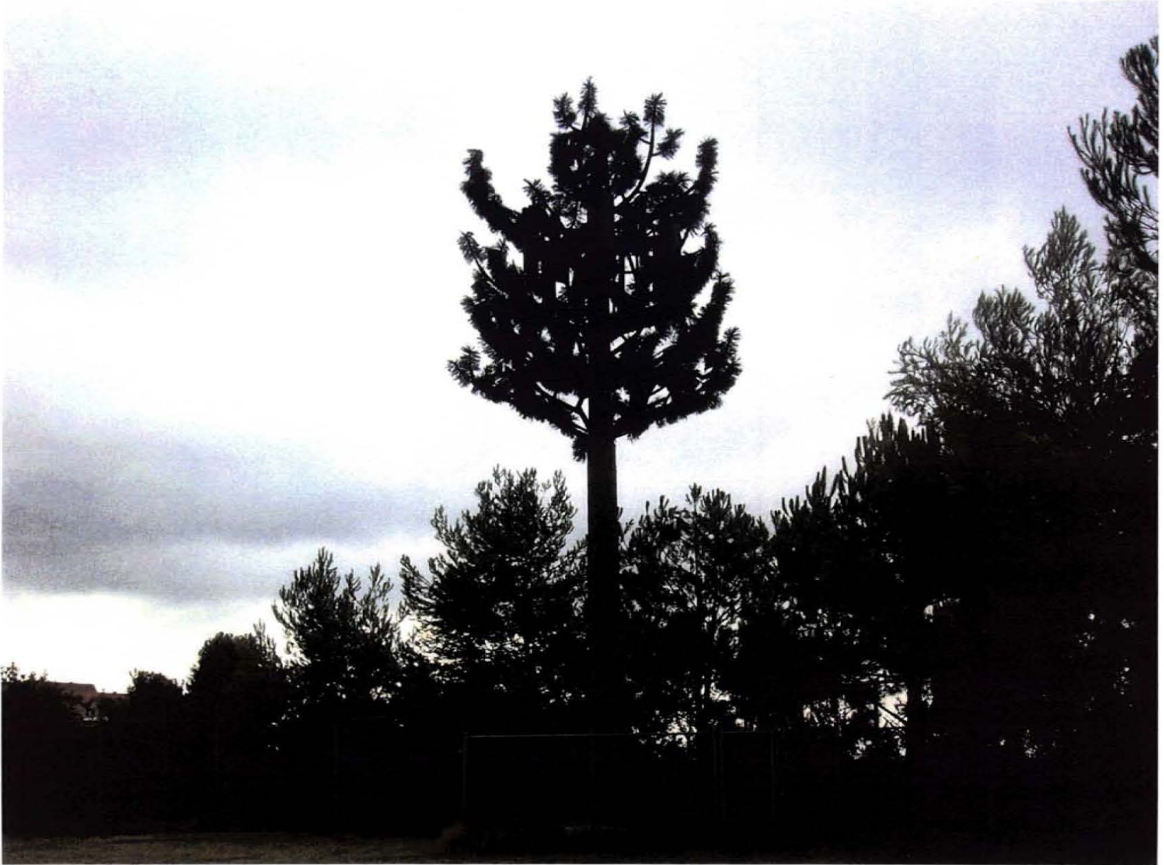
Existing Verizon monopine.
