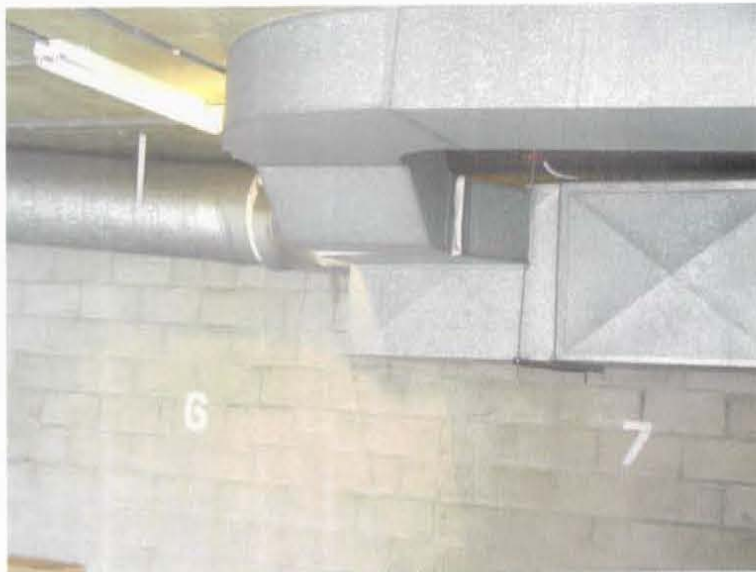
Part of garage exhaust system, which needs to be recommissioned.
