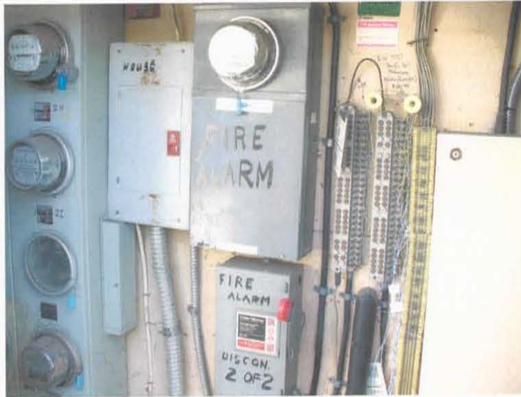
Electric service, including the Fire Alarm
