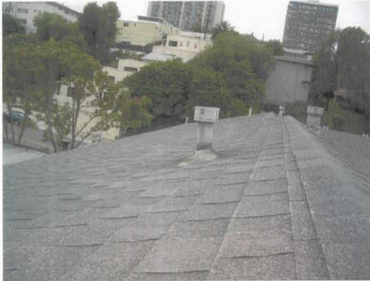
Light wear showing on the asphalt shingles.
